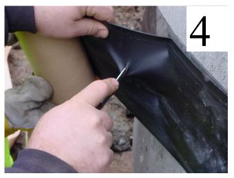
4. Cut excess material using a utility knife. Using a rubber mallet or hand held roller, firmly flatten the Gator Wrap® 360 degrees around joint.
