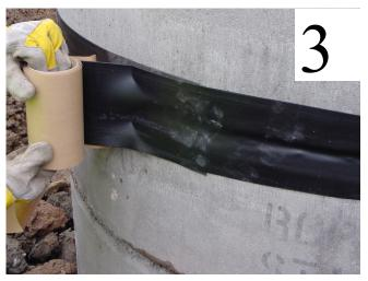
3. Seal the overlapping area with a 6" overlap. Be sure not to stretch material at the overlap area.
