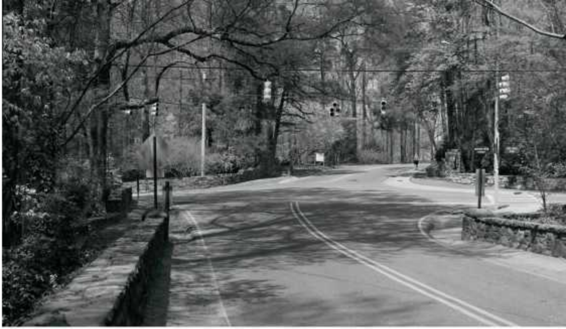
Overbrook Road Bridge and Entrance at Mountain Brook Parkway and Pine Ridge Road. Photograph by Jet Lowe, 2013. HALS No. AL-2-17.
