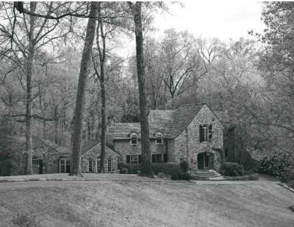
2737 Southwood Road, the Larkin House, a "Model Home" Sited on Its On Knoll. Photograph by Jet Lowe, 2013. HALS No. AL-2-13.
