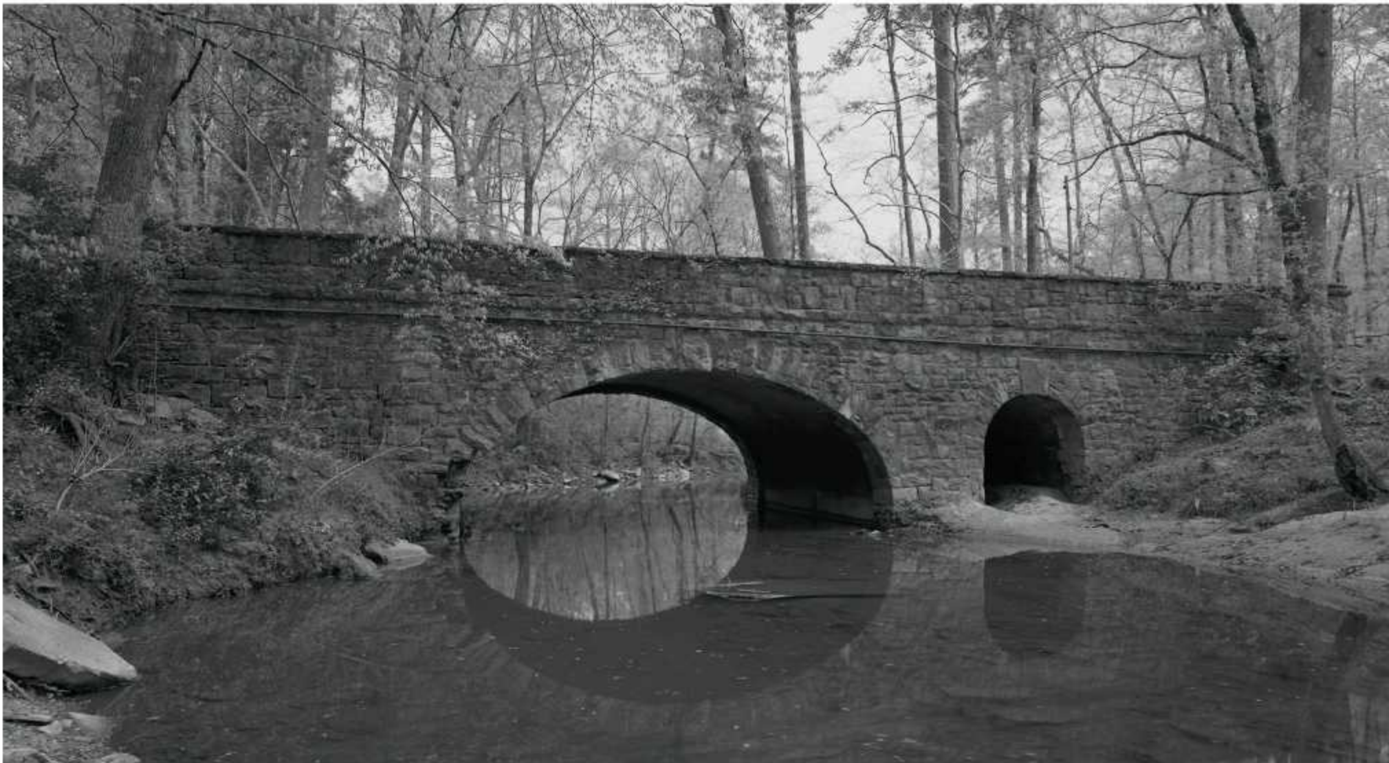
ABOVE: Overbrook Road Bridge. Photograph by Jet Lowe, 2013. HALS No. AL-2-18. Built in the style of early twentieth-century bridges that carried horse-drawn vehicles, the Overbrook Road Bridge is veneered with rough-cut, native stone. The bridge appears as if it belongs to the place. It does; its stone was quarried nearby. The archway, on the right , served horseback riders and pedestrians exploring the woodland trail.
