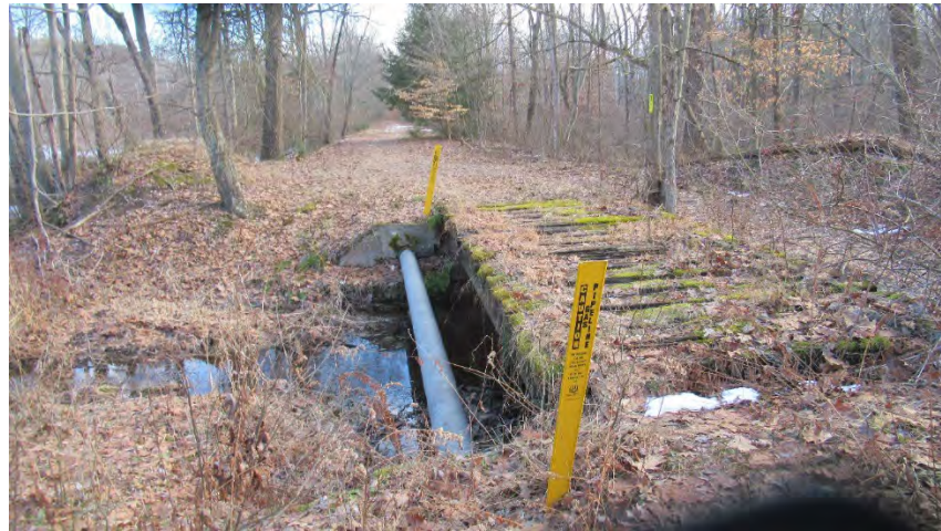
Figure 24: Bridge 4 – Snyderstown Girder Bridge in Snyderstown Borough
