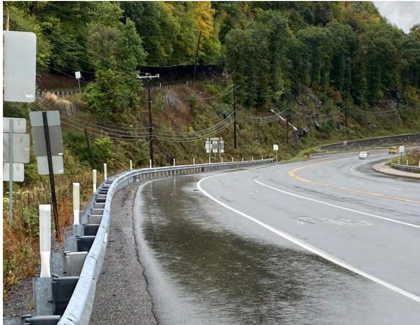
Figure 41: Corridor Alignment on SR 61 Facing North
