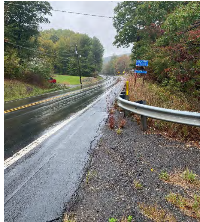
Figure 49: SR 901 & Upper Excelsior Road/Upper Main Street Intersection Westbound View
