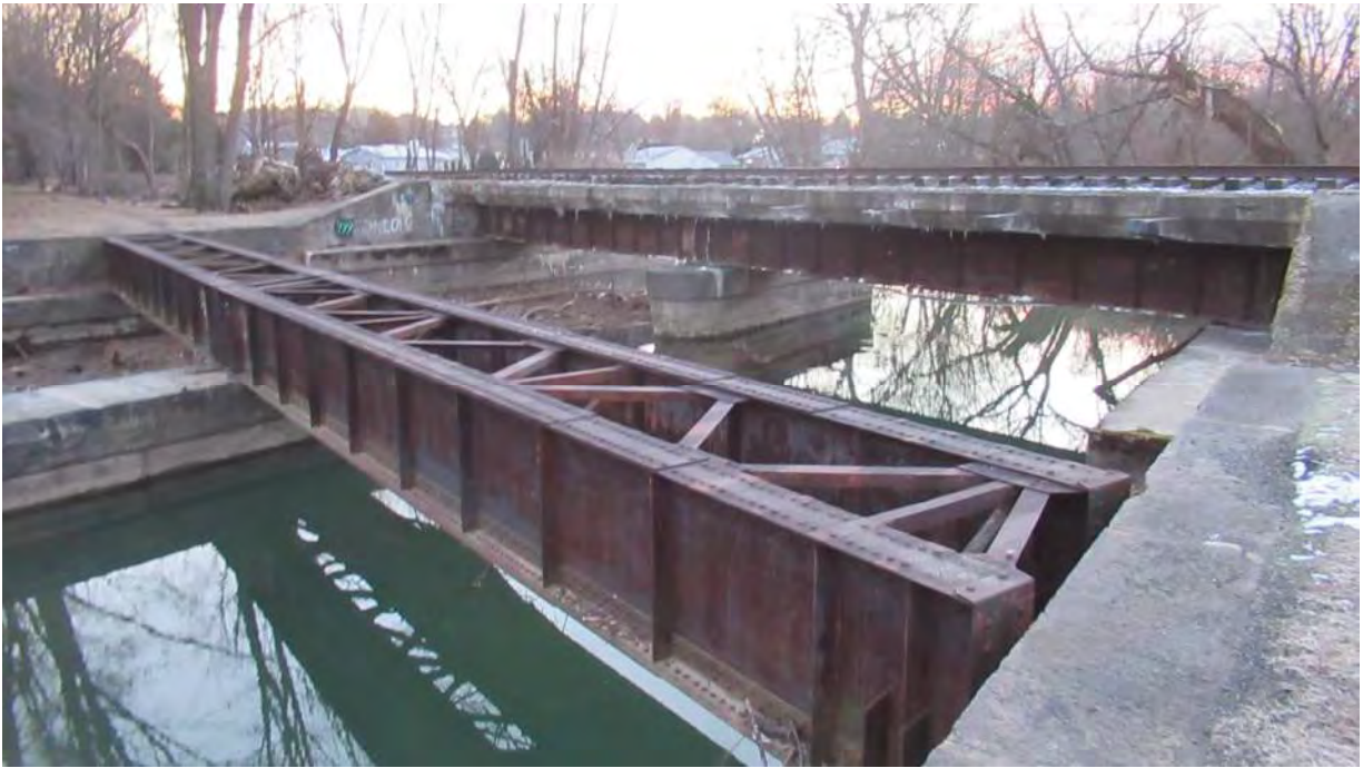
Photo3: View of subject structure in foreground and active railroad bridge adjacent to inspected structure.
