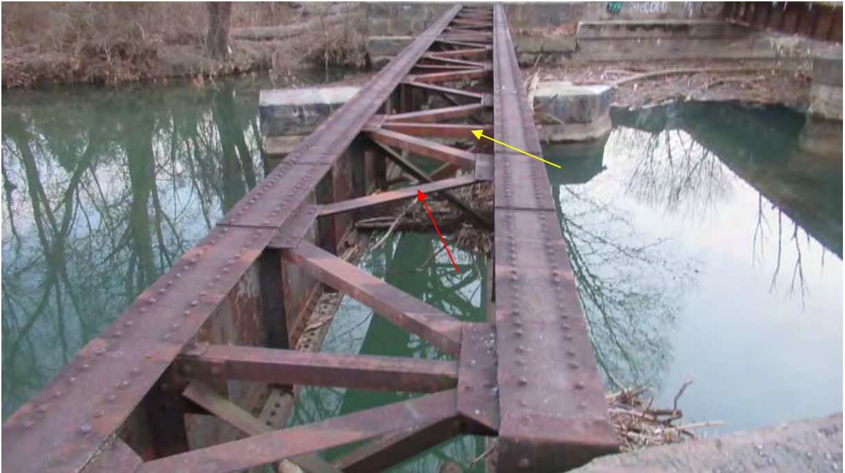
Photo 4: General view of the bracing for the two-girder system. Top flange lateral bracing (red arrow). Cross frame bracing (yellow arrow). Also note section loss of rivet heads.
