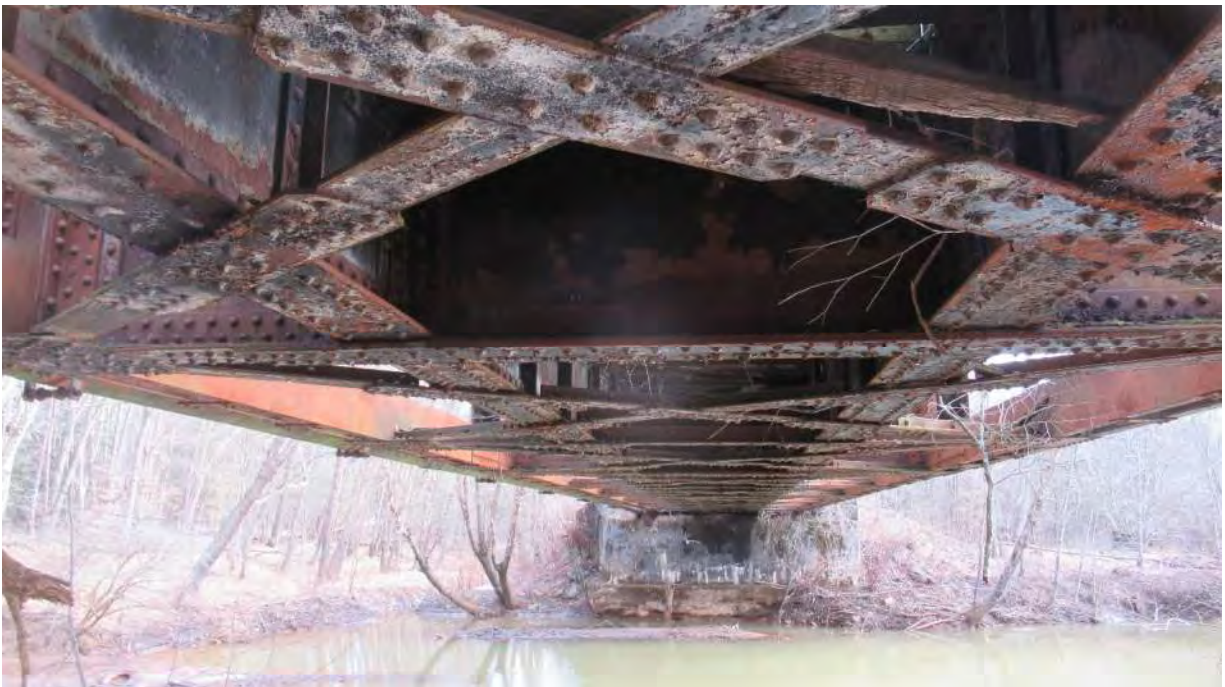
Photo 6: Lower lateral bracing for support.
