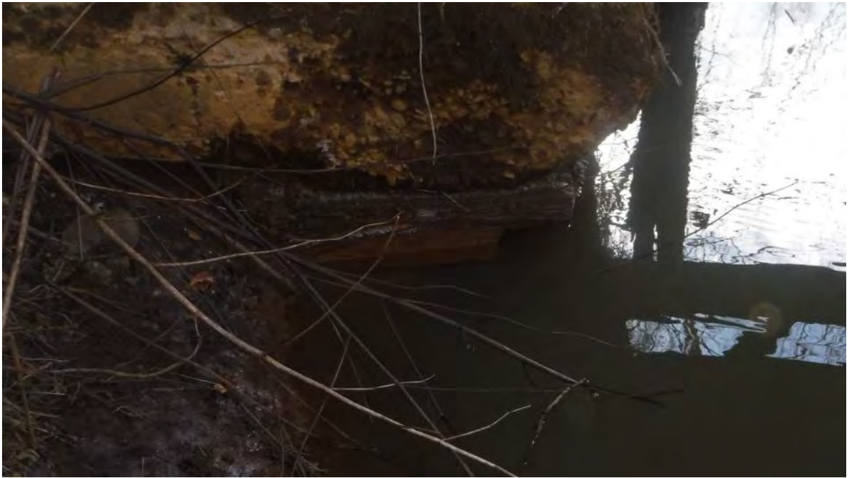
Photo 5: Exposed and undermined timber cribbing at East Abutment.
