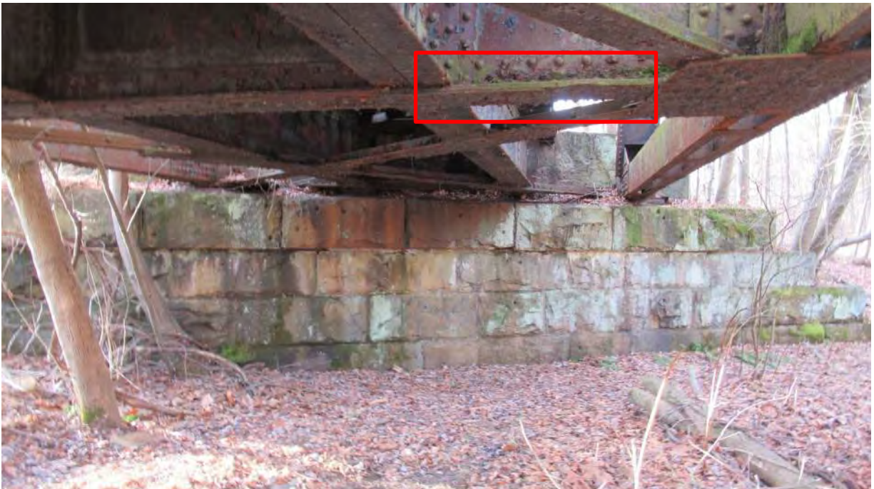
Photo 2: North abutment face. Note section loss to bottom of floorbeam.
