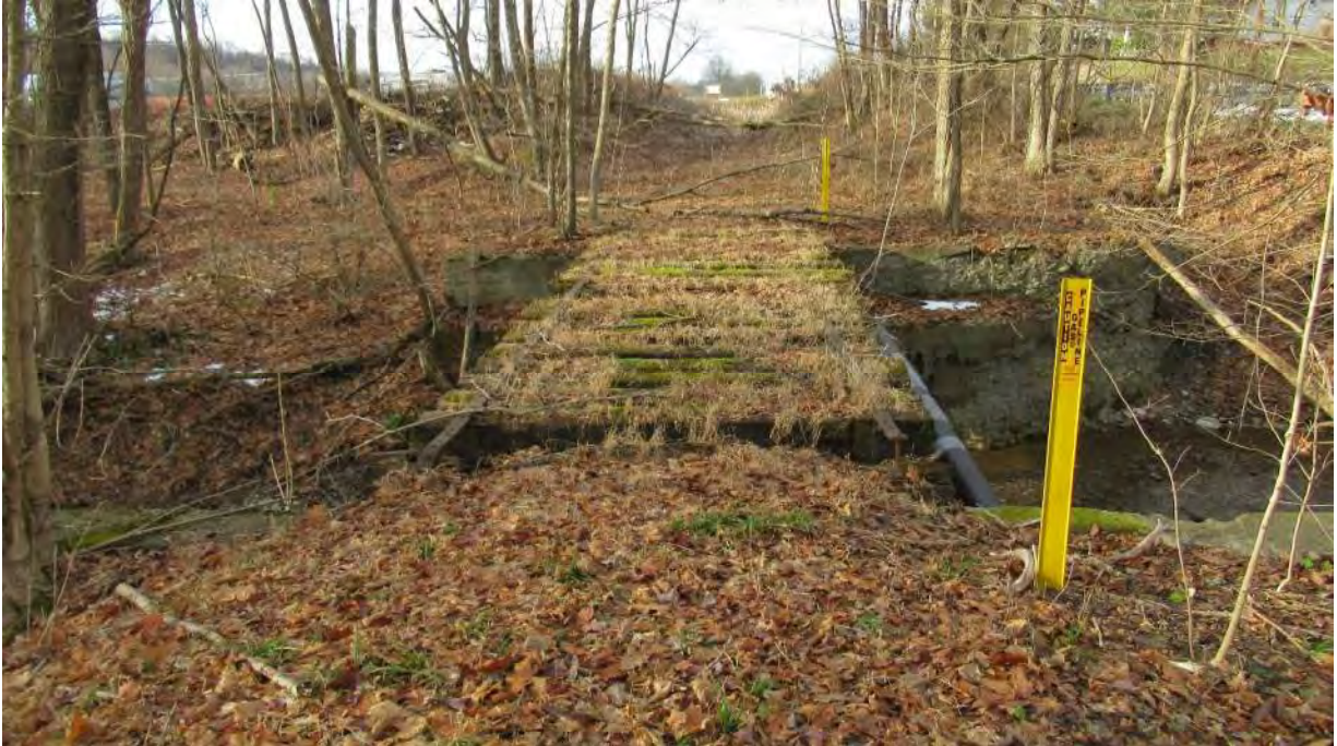
Photo 3: Overview of structure facing West. Note deterioration on West abutment.
