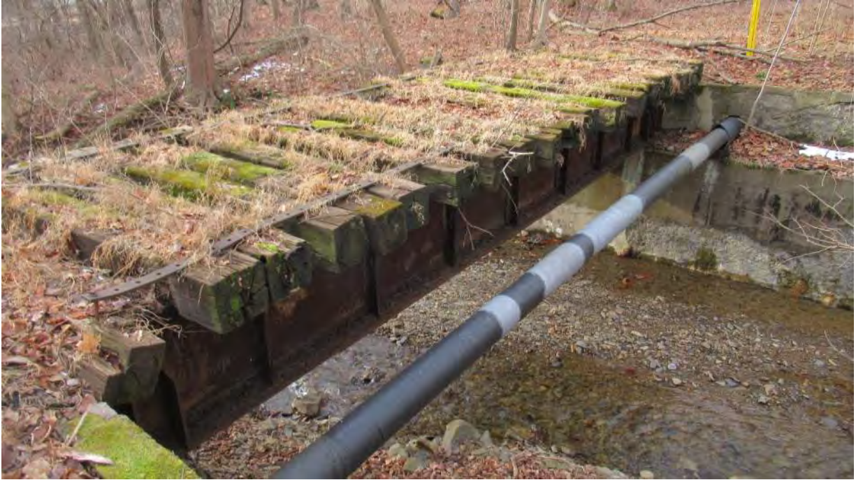
Photo 1: Overview of riveted plate girder bridge.
