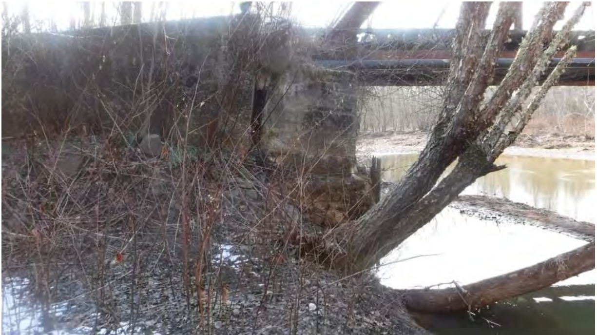
Photo 4: Note tilting of East side abutment. Tilt was measured at approximately 1” per foot.
