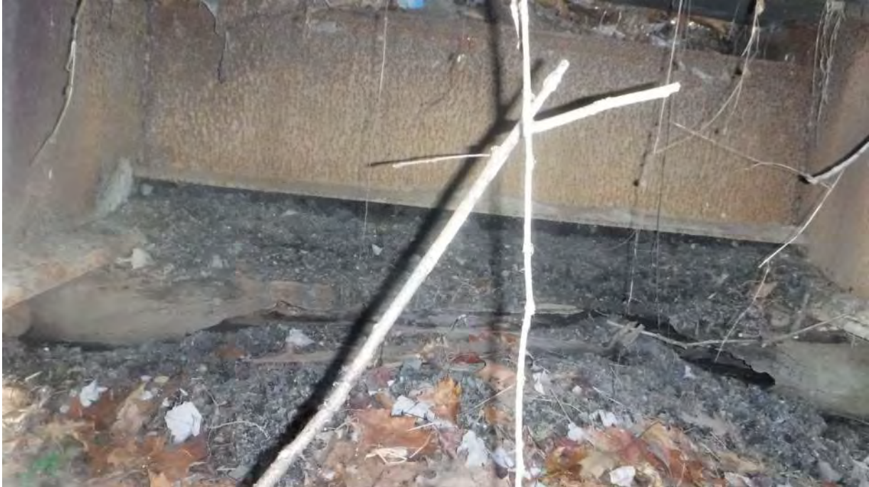
Photo 5: View of West abutment. Note severe deterioration of supporting timber.
