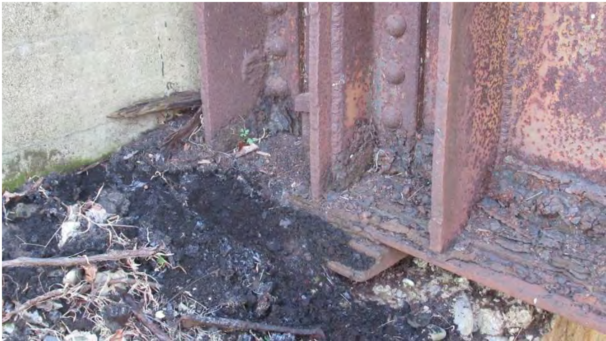
Photo 4: View of bearing area on East abutment with loss of support. Also note deterioration to top of bottom flange
