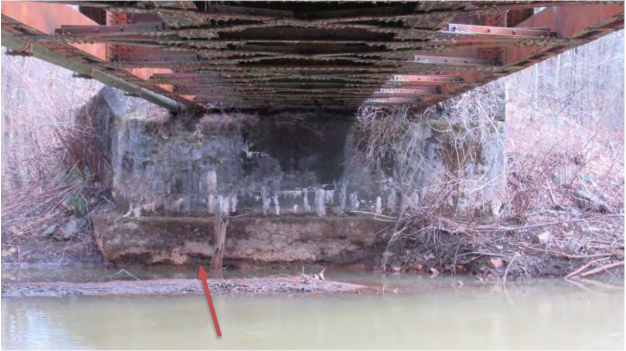
Photo 3: Abutment 2. Note spalling and undermining at footing.
