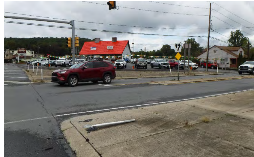
Figure 38: SR 61 & SR 487/Main Street Paxinos Intersection North View
