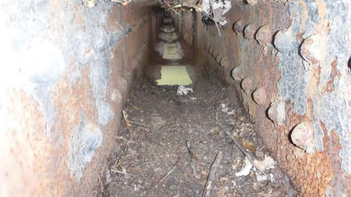
Photo 5: Heavy debris and severe section loss between lower cord truss members.
