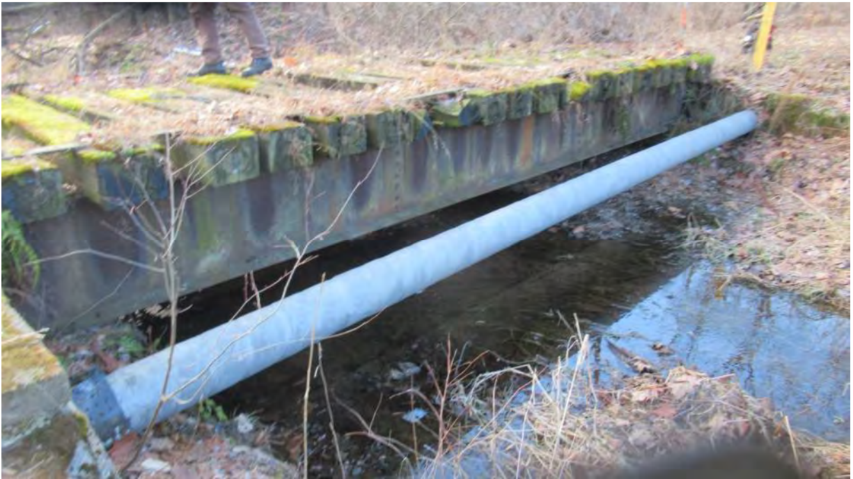
Photo 2: Self supported natural gas line.
