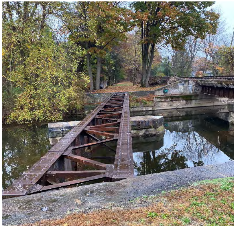
Figure 21: Bridge 1 – Upper Augusta Girder Bridge in Upper Augusta Township
