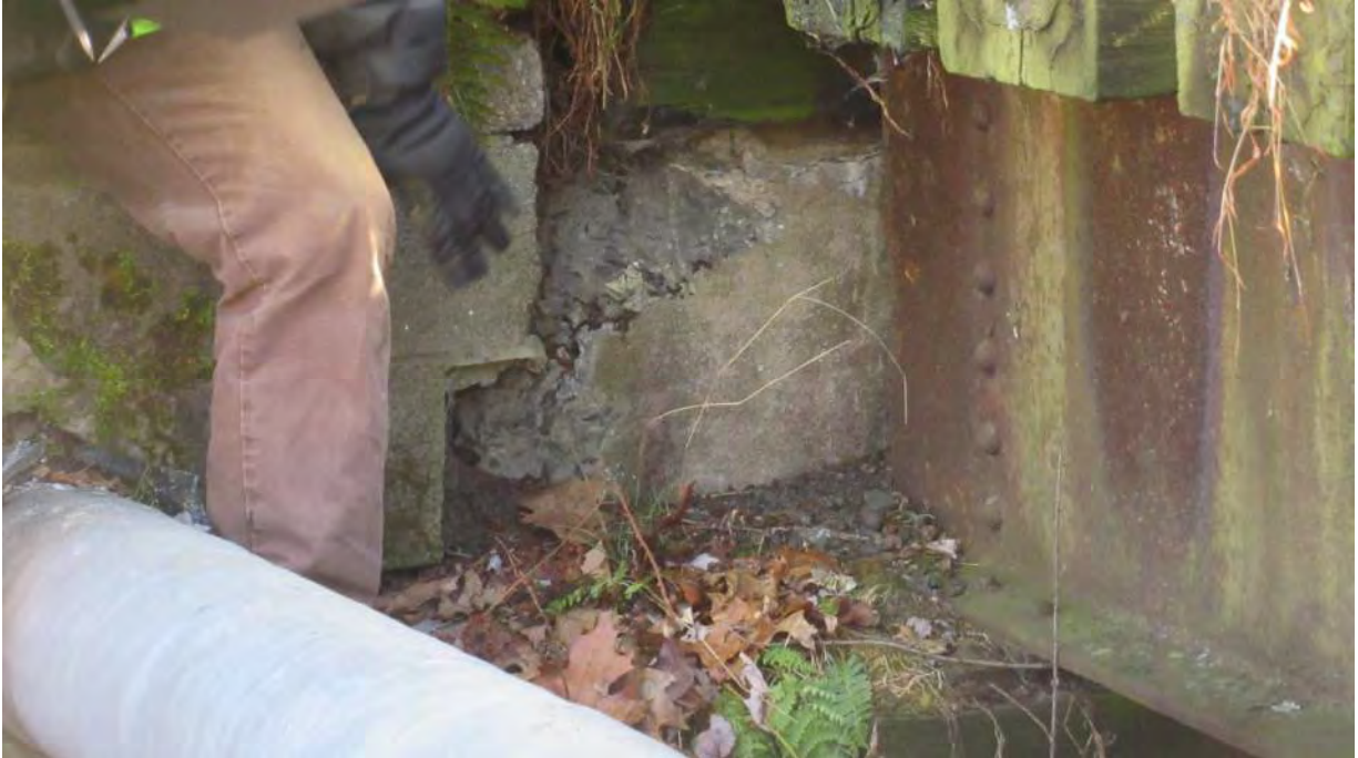
Photo 3: Concrete spalling at backwall.
