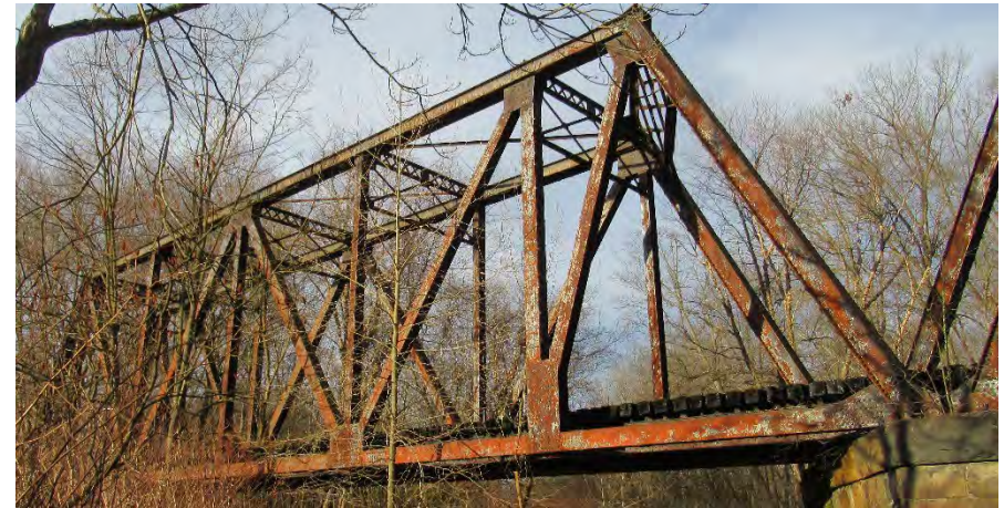
Figure 23: Bridge 5 – Shamokin Truss Bridge in Shamokin Township
