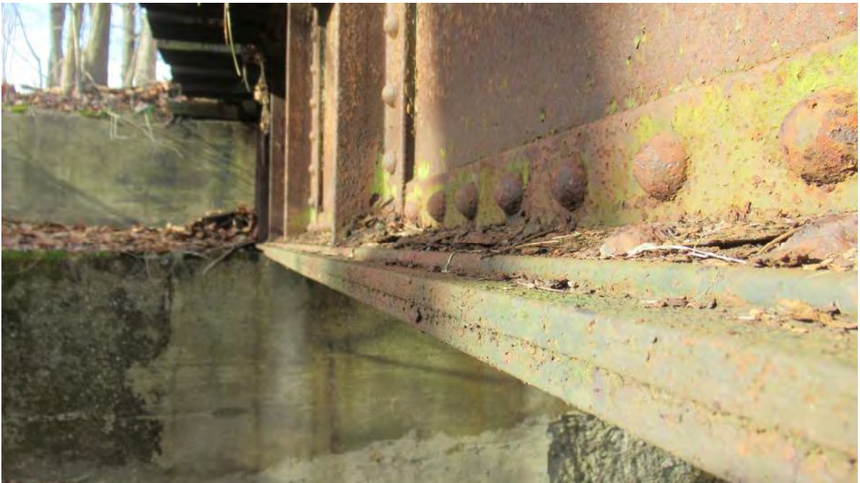
Photo 6: General view of the bottom flange of the built-up plate girder.
