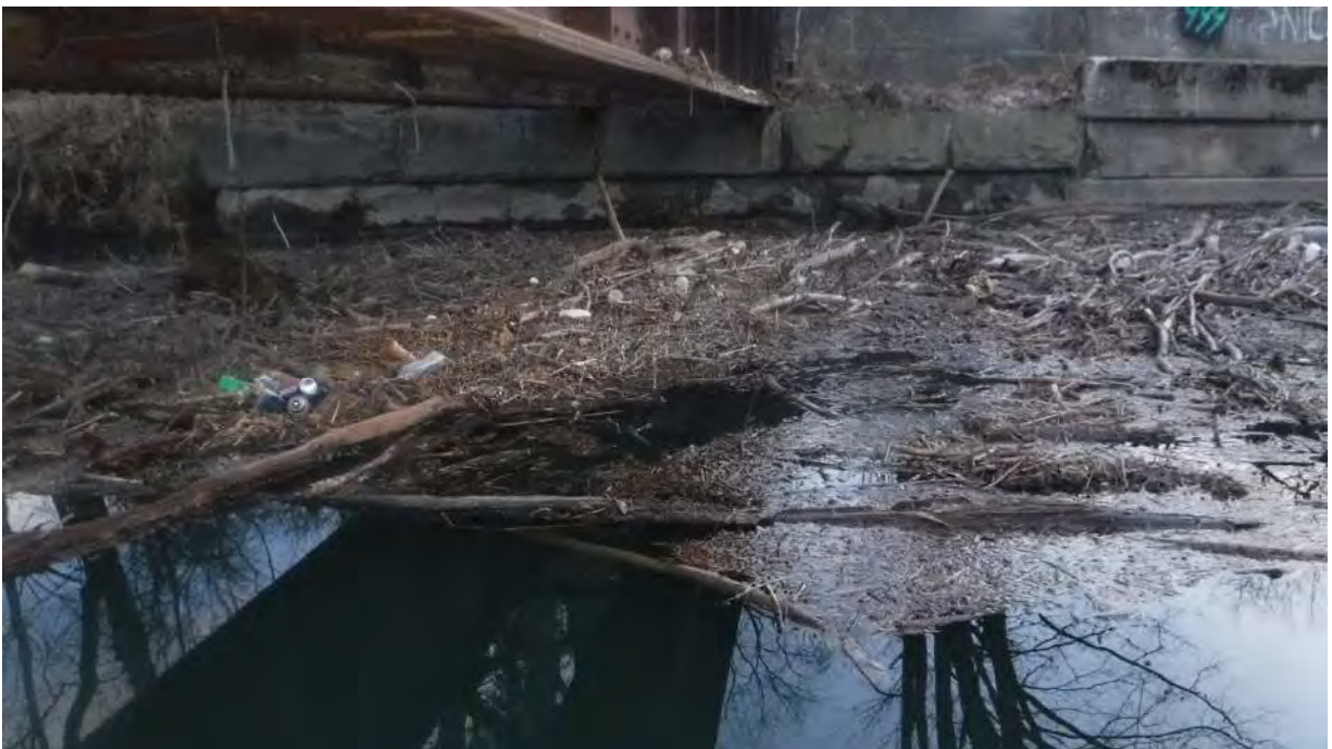
Photo 2: Debris observed in creek adjacent to East side abutment, superstructure, and substructure.
