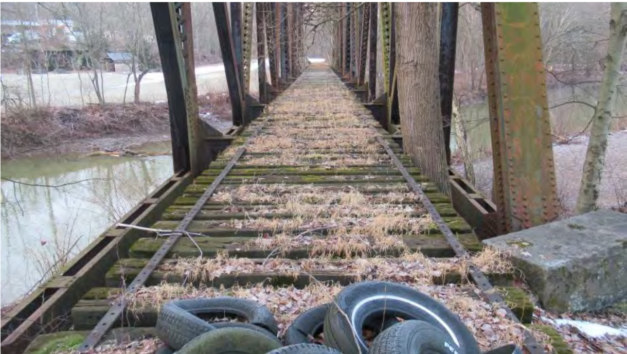
Photo 6: Looking South along centerline of structure. Note deterioration of timber and tree growing through superstructure.
