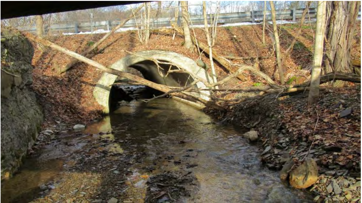
Photo 2: Upstream view from under bridge of concrete arch carrying SR 4012 over a tributary to Shamokin Creek.
