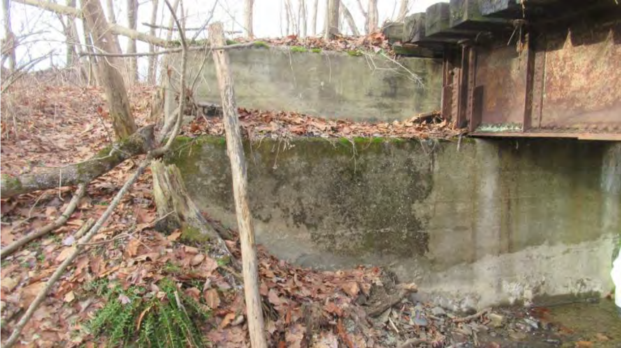
Photo 5: View of East abutment where only minor cracking is present.
