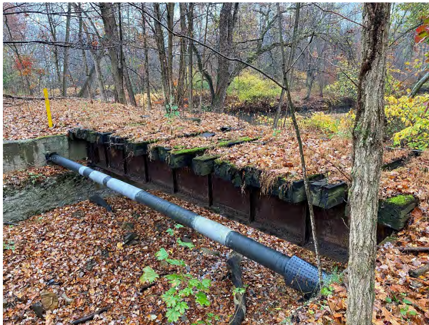
Figure 54: UGI Pipeline Adjacent to Bridge 3
