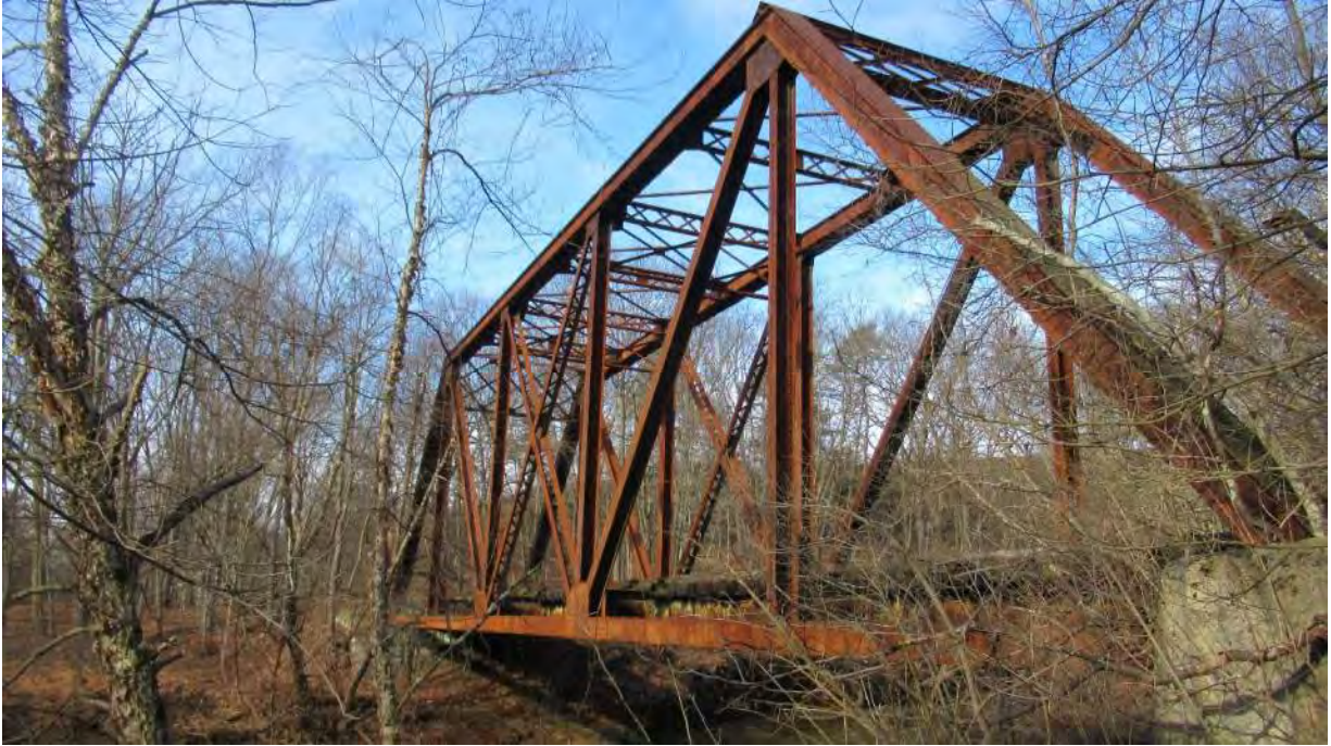
Photo 1: Overview of steel truss bridge.
