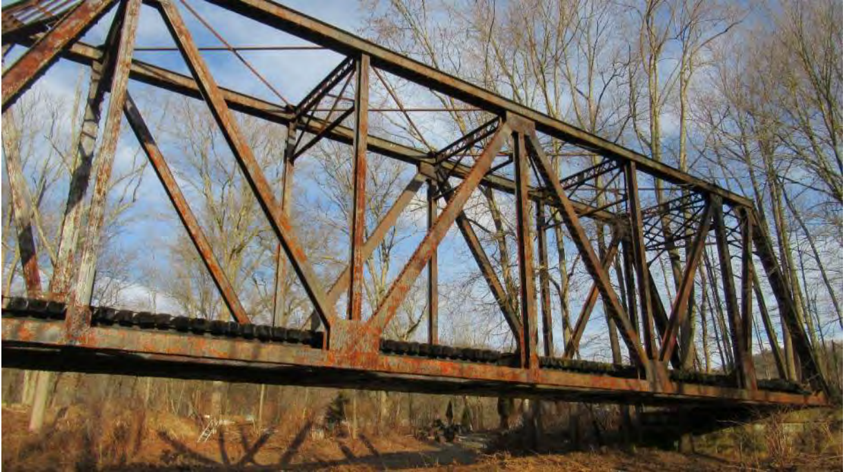
Photo 1: Span 1 of truss bridge looking West.
