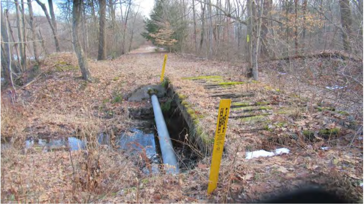
Photo 1: Overview of rolled steel girder bridge
