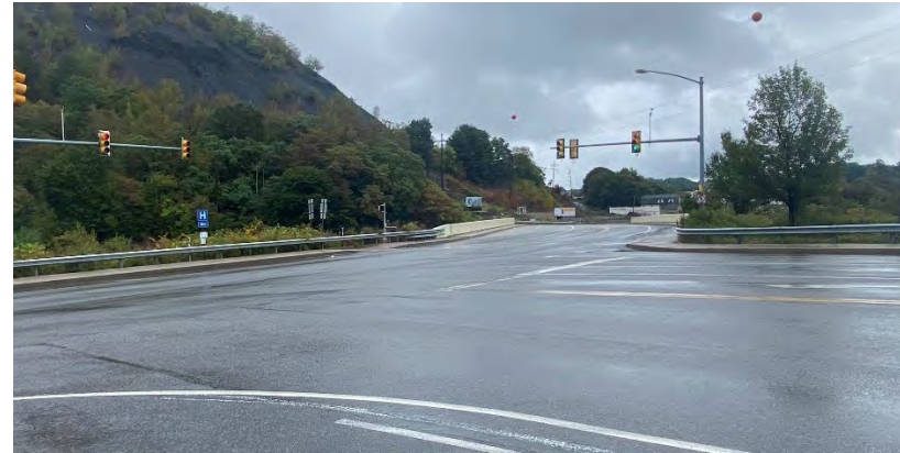
Figure 42: SR 61 & SR 225 Intersection Facing South
