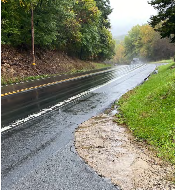
Figure 48: SR 901 & Upper Excelsior Road/Upper Main Street Intersection Eastbound View
