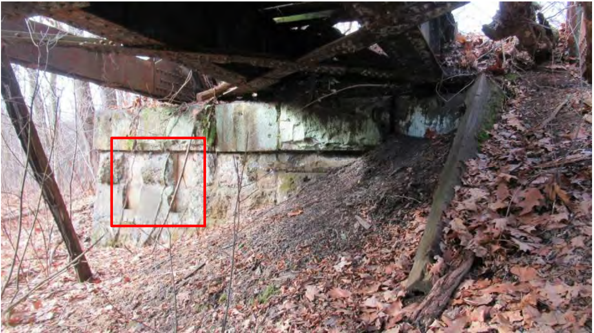
Photo 2: West Abutment. Note slots, and soil falling over the face of abutment and buried backwall/bearings.
