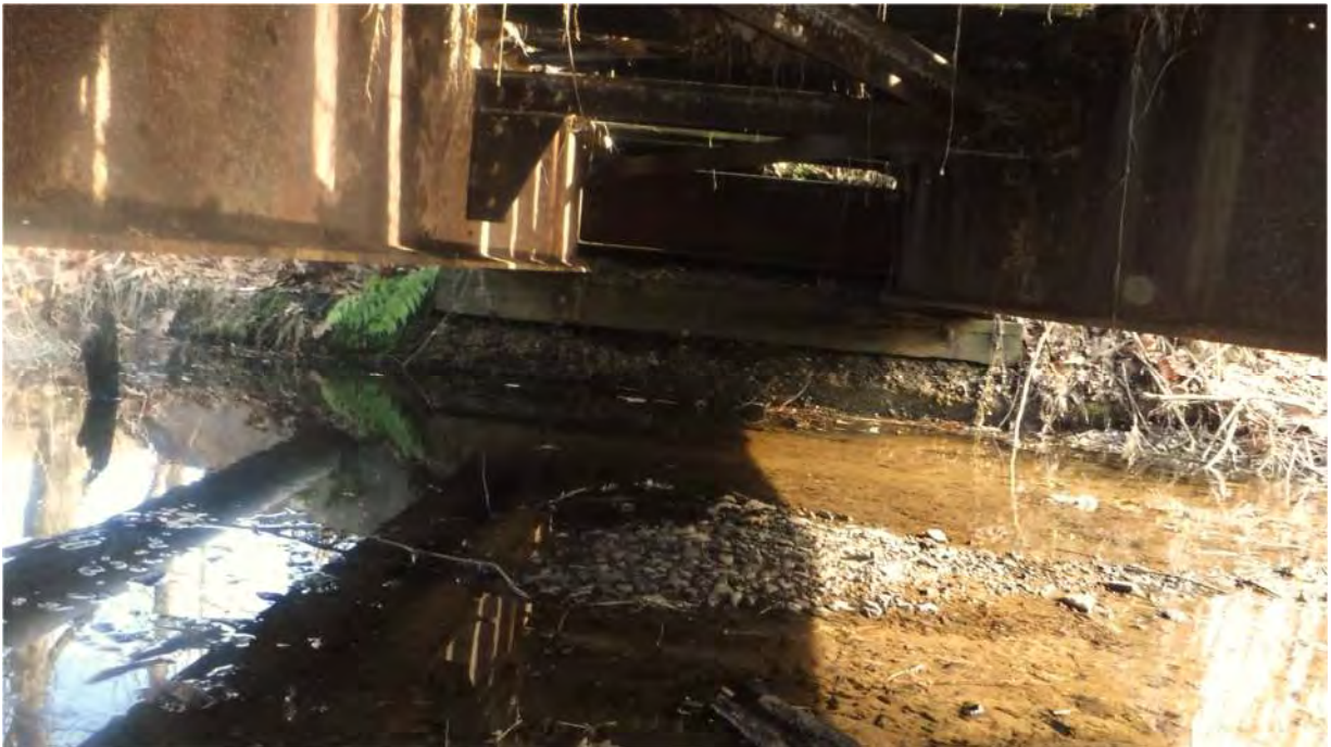
Photo 4: View of East abutment. Note deteriorated timber member supported by spalled concrete.
