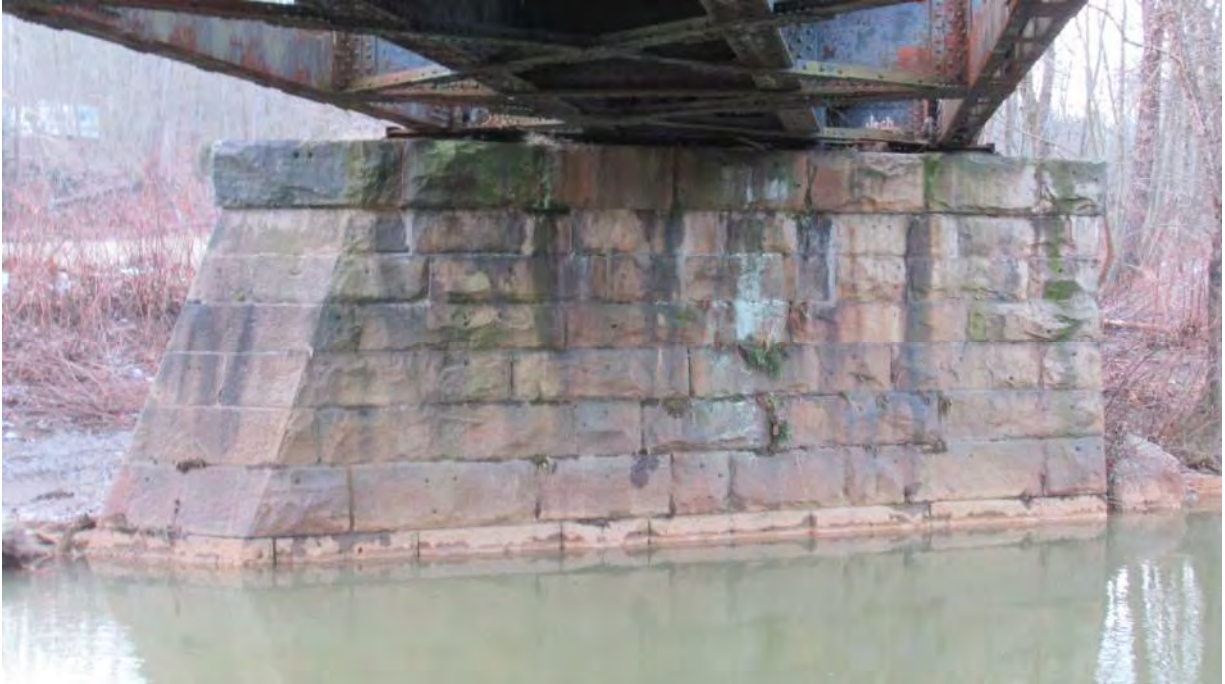
Photo 3: Span 1 side of stone masonry pier face.
