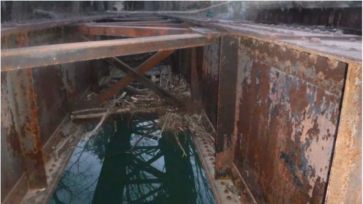
Photo 1: Interior view of riveted plate girders. Note flood debris trapped on diaphragms and vertical stiffeners on the interior of the structure.
