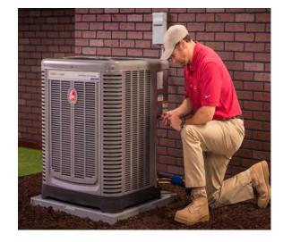
When an Air Conditioner coil becomes fouled with dirt and grime, it cannot provide adequate cooling. This requires more electricity and will increase the cost of operation. In fact, the energy consumption of dirty equipment can be as much as 37% more than clean equipment.
