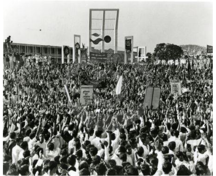
1963-71 Third Shaheed Minar. February 21, 1971 Designed by sculptor Hamidur Rahman the construction of third Shaheed Minar began in 1957. It was inaugurated on February 21, 1963.
