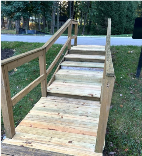
Boardwalk stairs repairs and renovation
