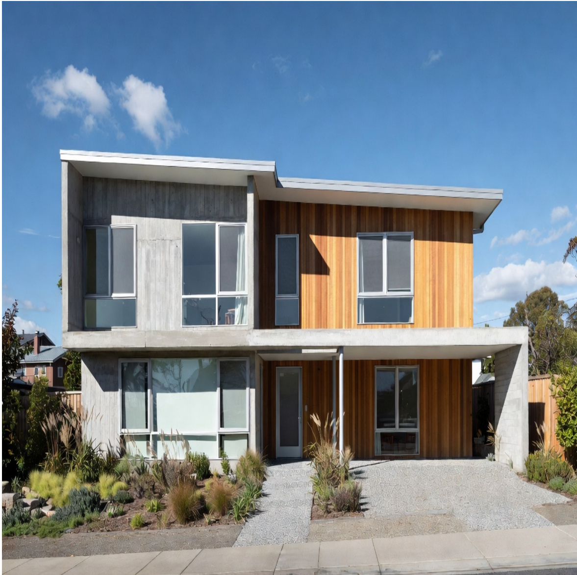
Concept B — Hybrid concrete and timber-clad residence. Full-height concrete perimeter walls at ground level with upper-level timber cladding for warmth and reduced thermal bridging.
