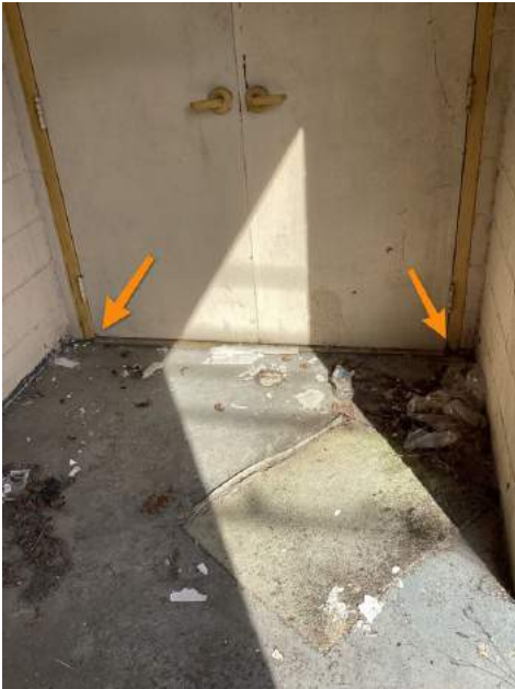
Rear of Structure
