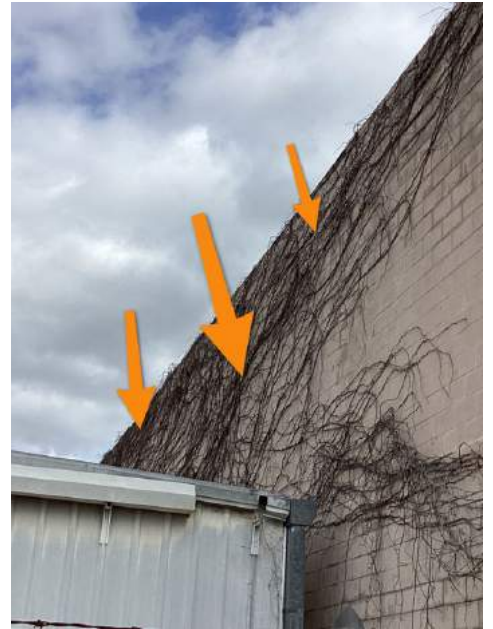
Right Side of Structure
