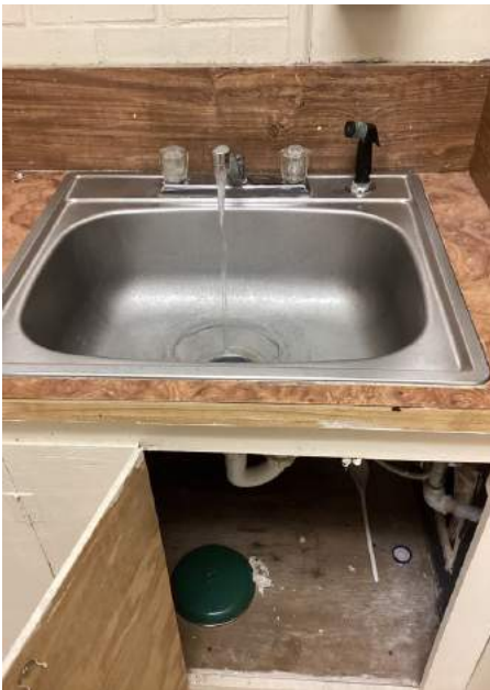
Middle Conference Room Sink
