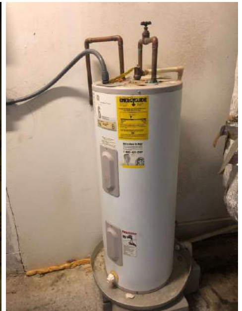
Upstairs HVAC Room
