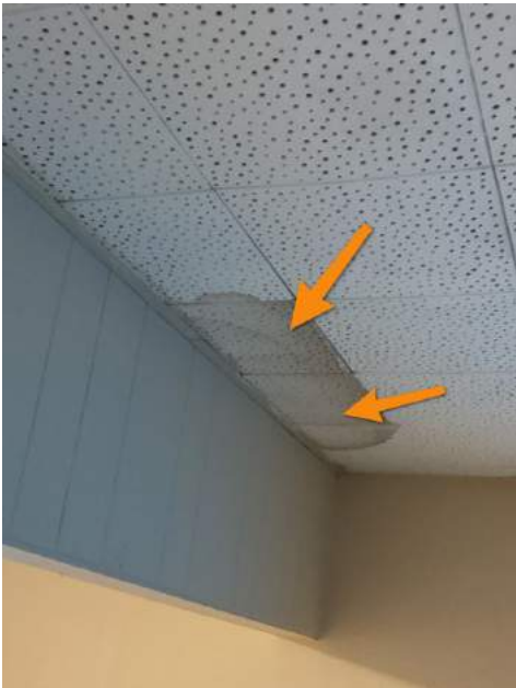
Left Hallway Office
