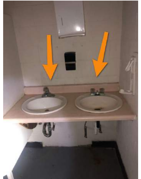
Men's Downstairs Bathroom
