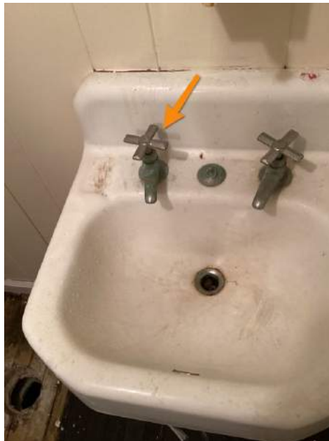
Upstairs Office Bathroom
