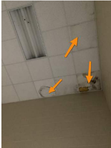
Interior Stairwell Ceiling
