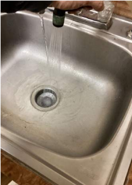
Middle Conference Room Sink
