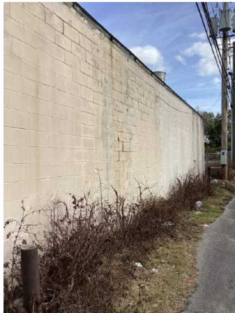
Rear of Structure
