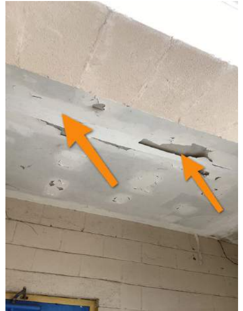
Rear Entry Ceiling
