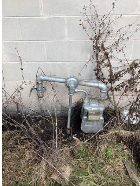
Rear of Structure
