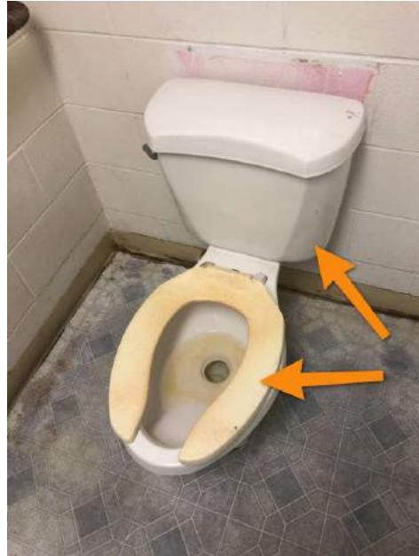
Downstairs Women's Bathroom
