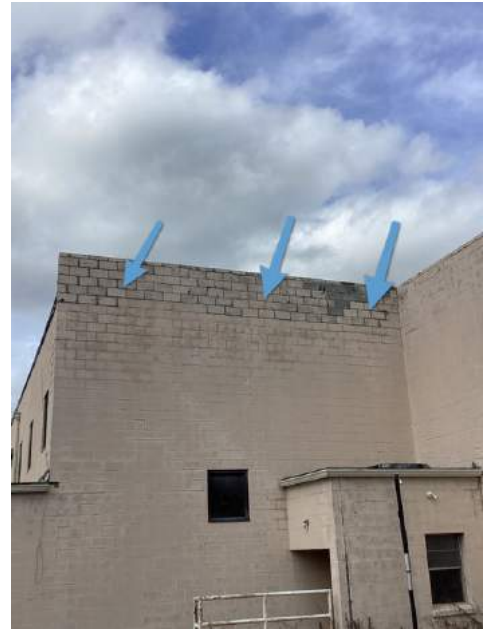
Rear of Structure
