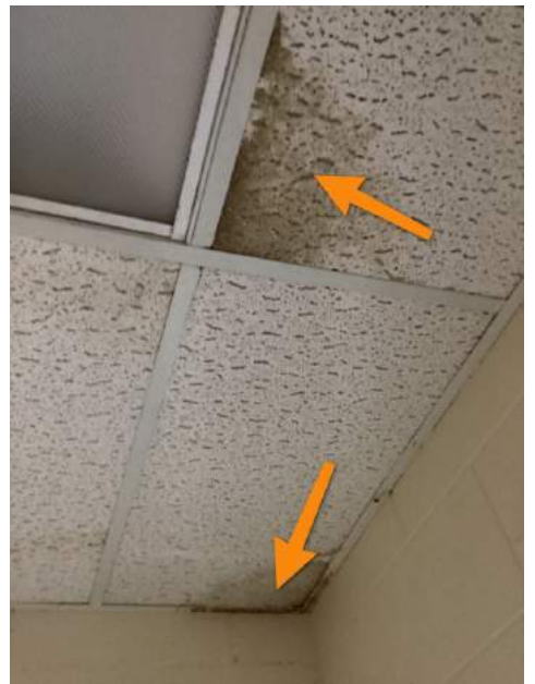
Downstairs Classroom Bathroom
