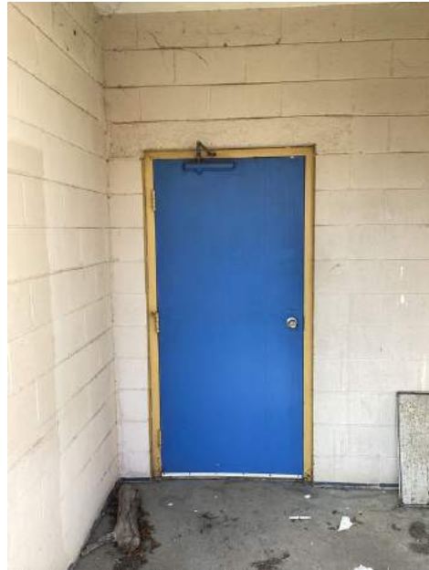
Rear of Structure
