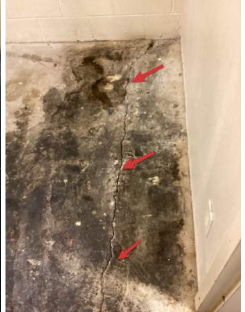
Upstairs Hallway Storage Room
