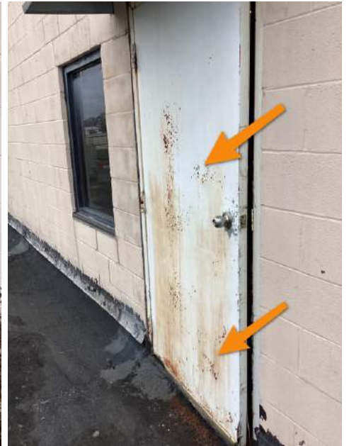
2nd Floor Exterior Door
