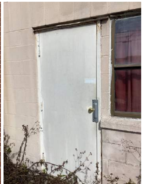
Rear of Structure
