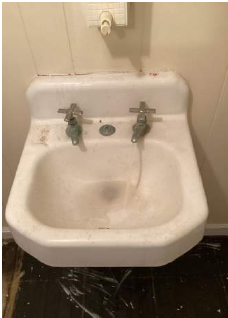
Upstairs Office Bathroom
