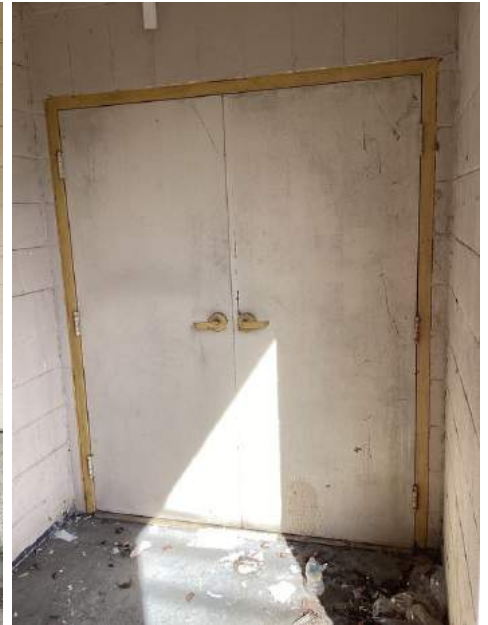
Rear of Structure Bathrooms
