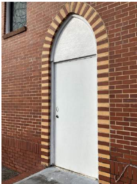
Left Side of Structure
