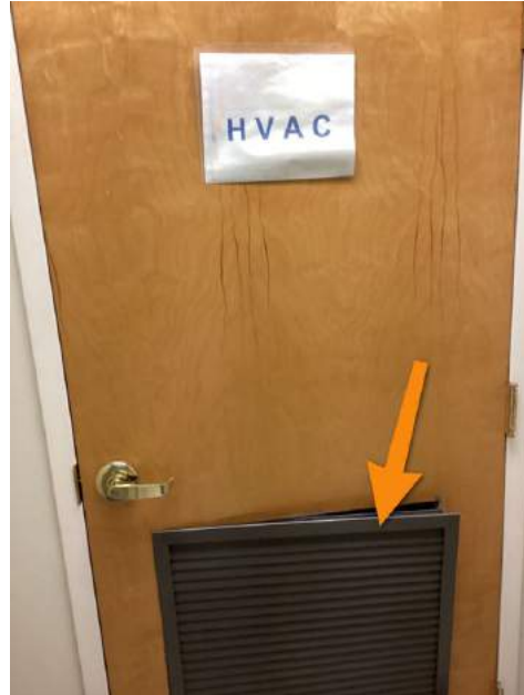
Upstairs HVAC Room
