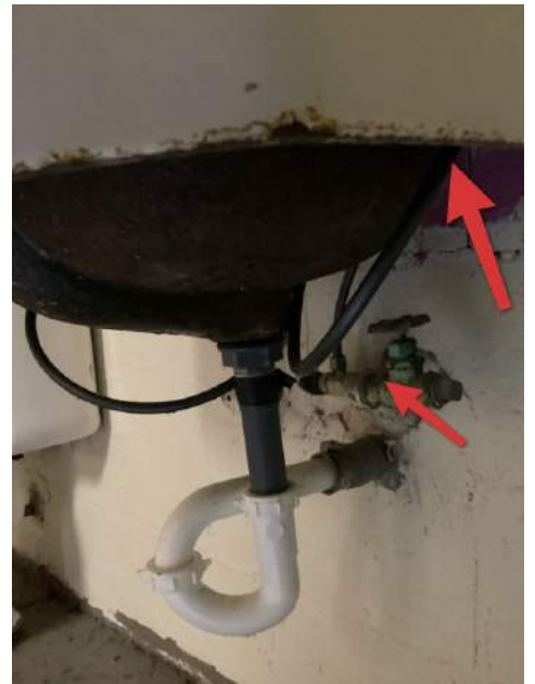
Downstairs Classroom Sink
