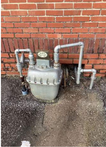
Left Side of Structure
