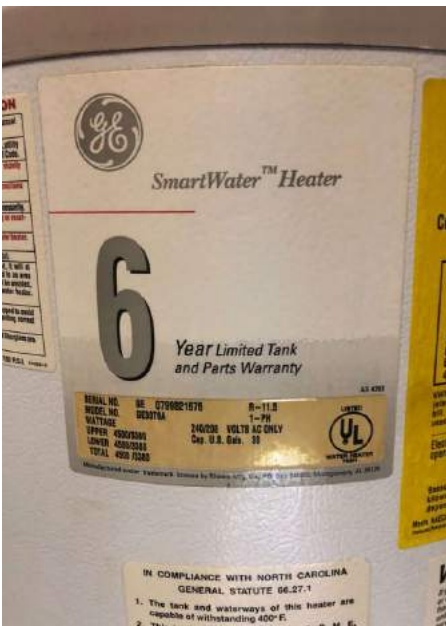
Upstairs HVAC Room
