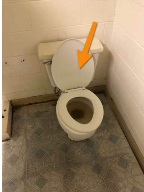
Downstairs Women's Bathroom
