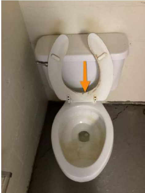
Downstairs Classroom Bathroom
