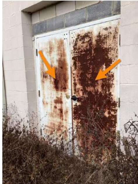
Rear of Structure
