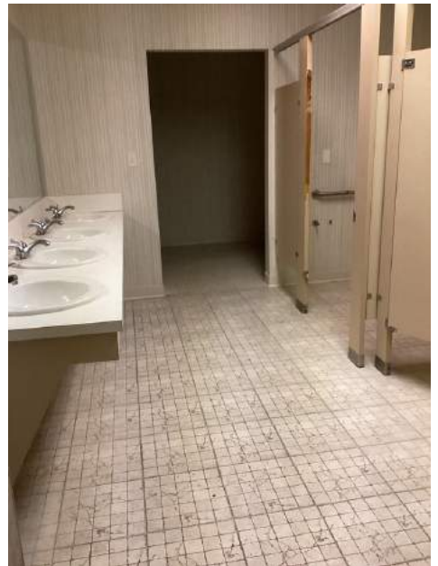
Upstairs Men's Bathroom
