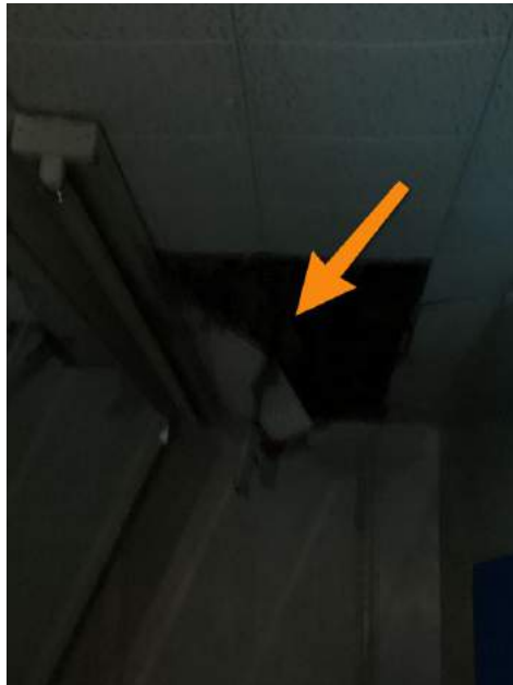
Ceiling Over Baptism Vault
