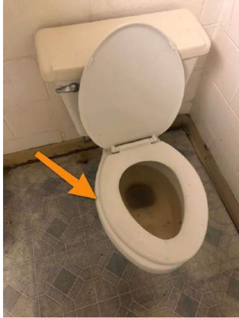
Downstairs Women's Bathroom
