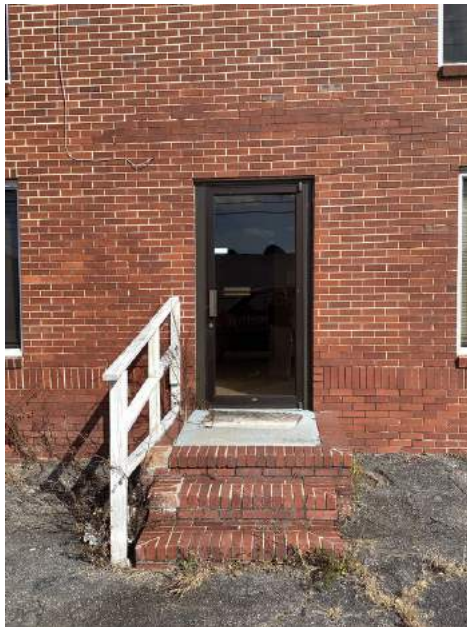
Rear of Structure
