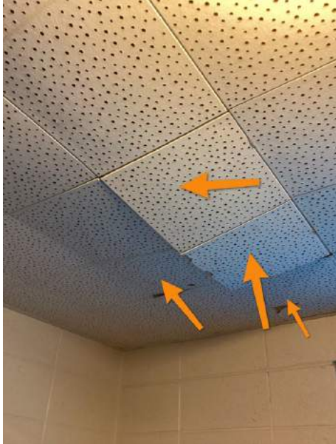
Left Side Hallway Room
