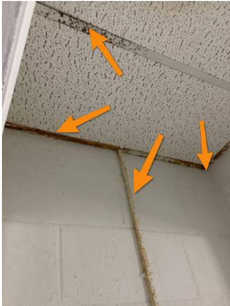
Downstairs Classroom Bathroom
