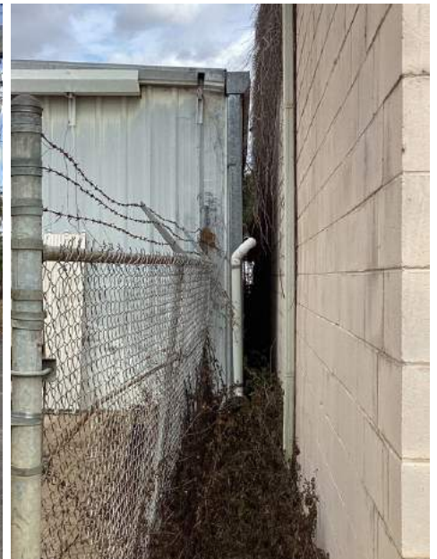
Right Side of Structure
