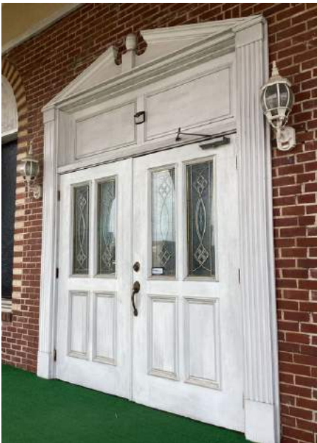
Main Entry Doors
