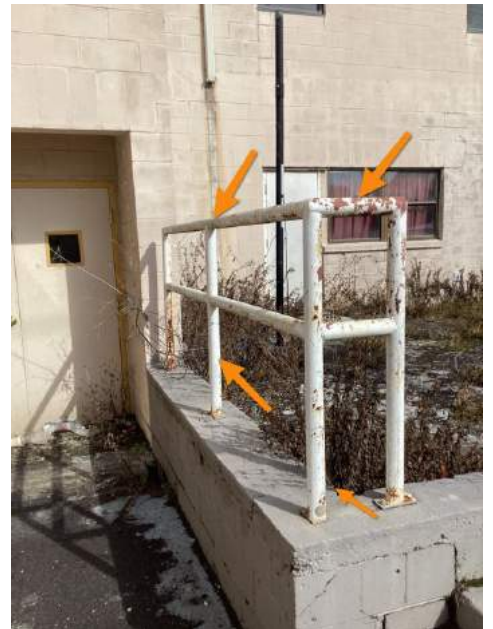
Rear of Structure
