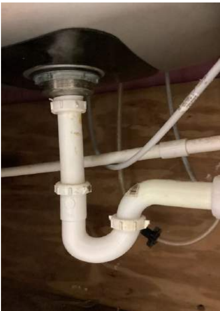
Middle Conference Room Sink
