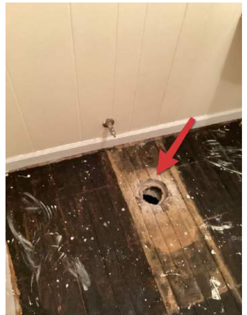
Upstairs Office Bathroom
