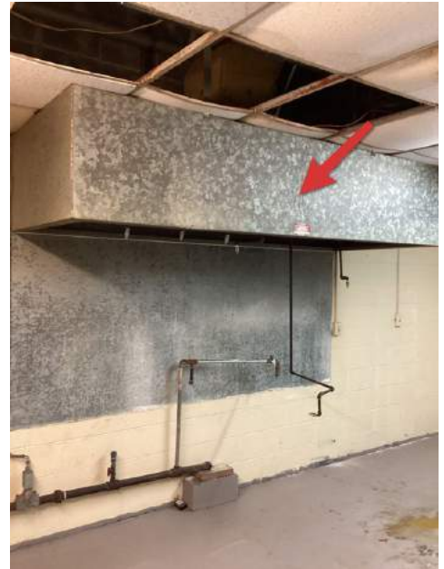
Cafeteria Hood Not Inspected
