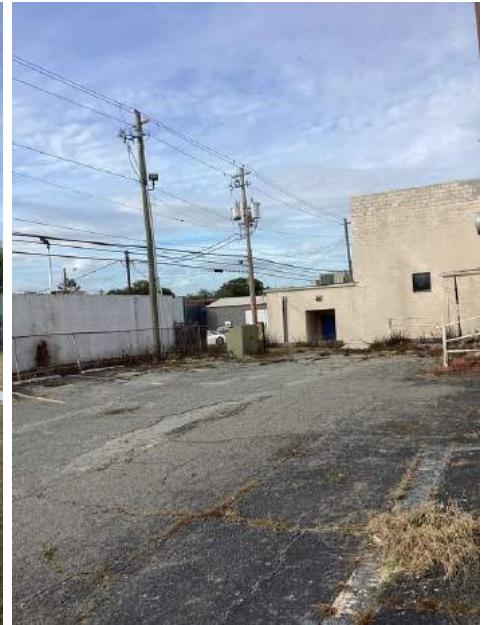
Rear of Structure In
