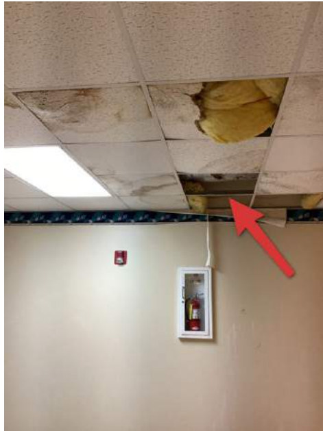
Upstairs Classroom Hallway
