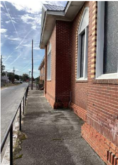
Left Side of Structure
