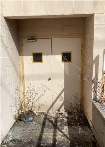
Rear of Structure
