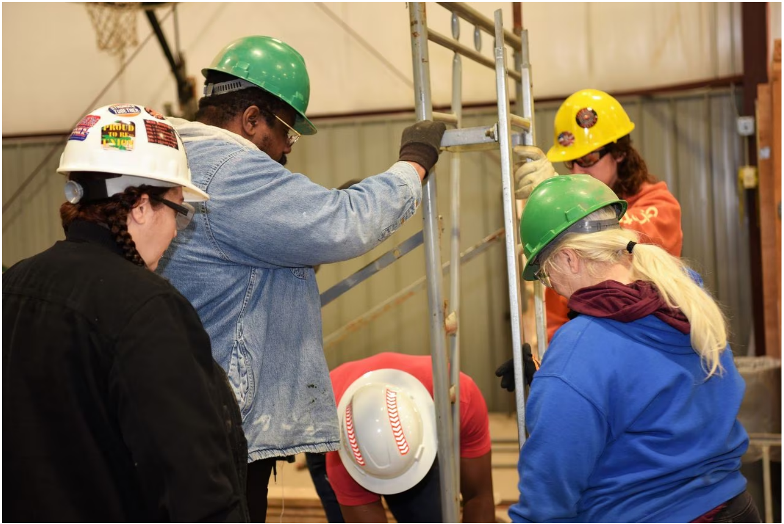
Apprentices learn how to erect scaffolding at the Upstate New York Laborers Training Center in Oswego. (Provided photo)
