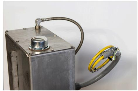
The Thermocouple sensor (A99) is mounted and wired to the reservoir. It will be the gray sheathed wire and labeled for connection to the TB3 terminal in the A421 control. Refer to A421 control manual for specifics. The A99 sensor is non-polar and either wire can be connected to the (-)COM or (+)SEN terminal.
