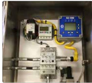
Pellet mill lubrication is critical in maintaining roll longevity. Excessive pellet mill grease both contaminates product and increases operational costs. GOLD has a feedback control solution:
