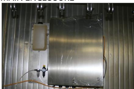
**Available Modes:** Manual Timed - Push button "ON", will terminate lubrication cycle at end of programmed timer duration.
