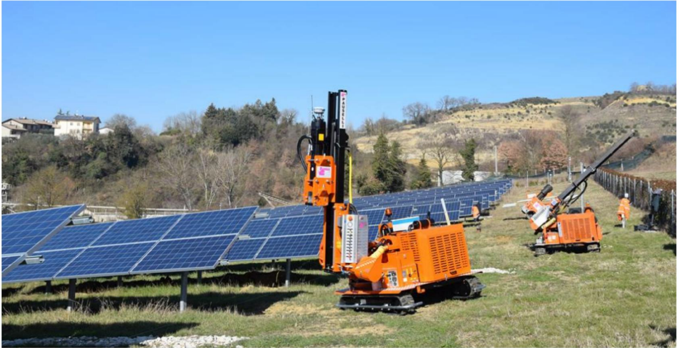
Image 1: Typical GPS Solar Farm Pile Driver
