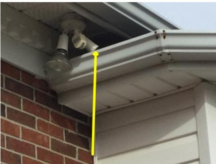
Missing bulb, recommend moving fixture so bulb will not over hang roof and possibly cause a fire.
