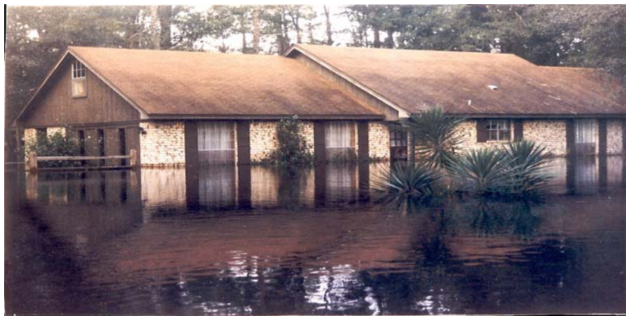
October 1994 Located in Zone X... Area least likely to flood 22 inches of water inside
