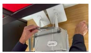
9. Bring the box to the pole mounting location. Open the hose clamp and install on post
