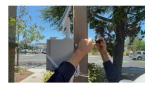
11. Align the solar panels to face south. Note, solar panels should receive ~4-5 hours of sun a day for optimum working conditions. If the camera location is in a shaded area, unscrew the solar mounts and mount them into the sun. The cameras come up ~ 6 ft of cable for flexibility
