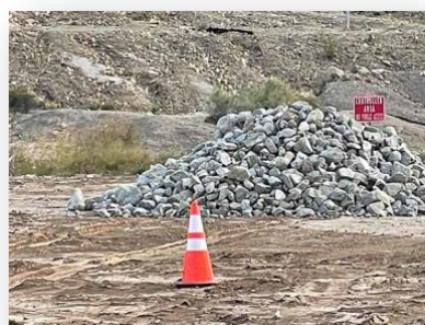
The first of many piles of rocks.
