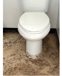
Newly remodeled bathrooms flooded as well.
