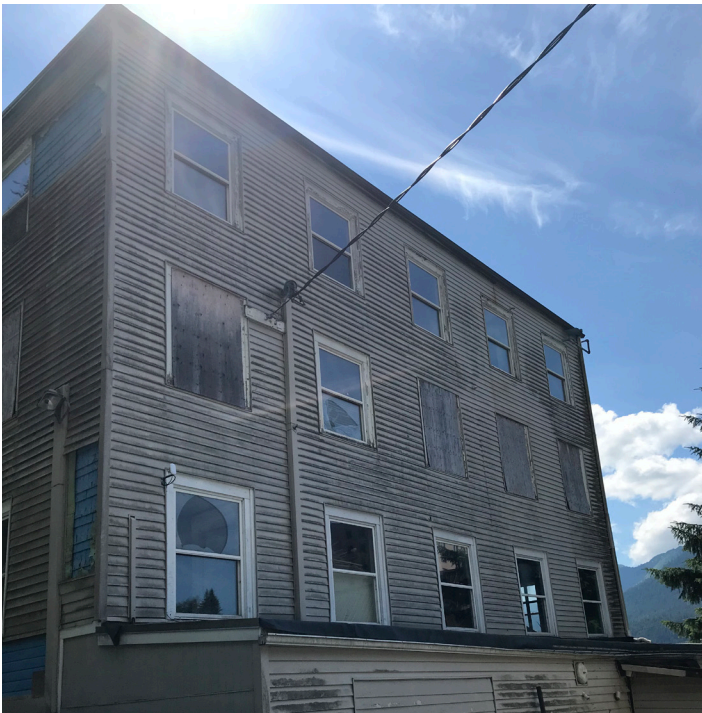
Main south entry detail image. Some water damage at grade that needs repair. Door does not appear original, however, is made similar to historic.
