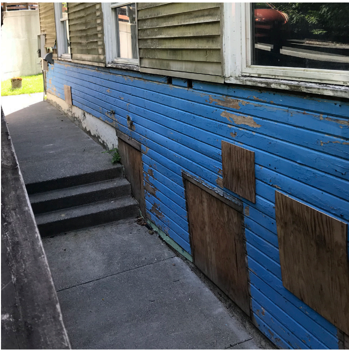
Bracing framing at corner exterior walls. Some interior partition walls have similar brace frame which are called out in the drawings. Header details uses bracing as well and all appear in good condition.
