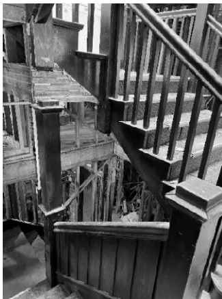
Figure 8 - No connections from column to stair landing.
