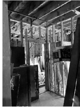
Figure 22 - King studs are discontinuous on either side of the door opening.
