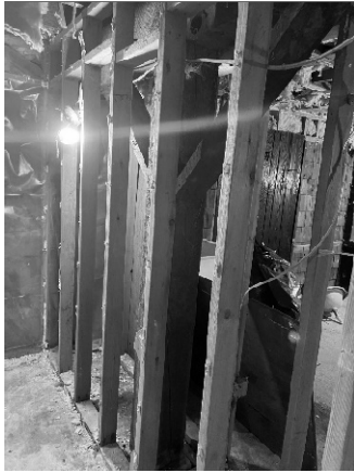
Figure 10 - Knee braces to transfer lateral loads.
