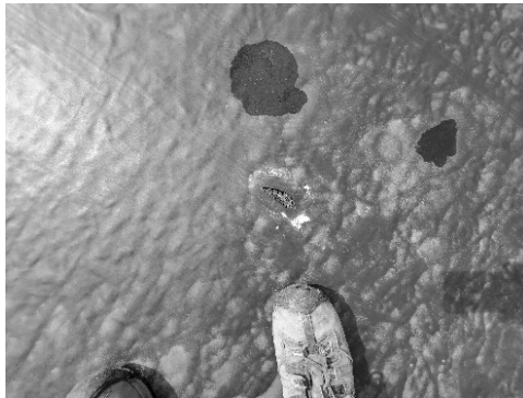
Figure 51 - There are a few small holes in the roof, which allow water to infiltrate.
