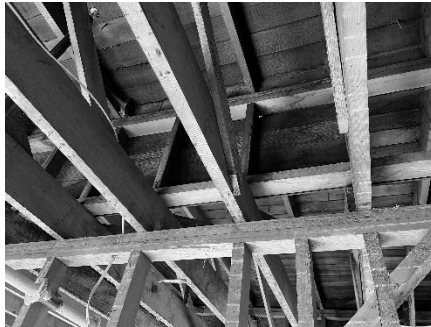
Figure 2 - Roof trusses do not have diagonal bracing from the roof diaphragm to the shearwall.
