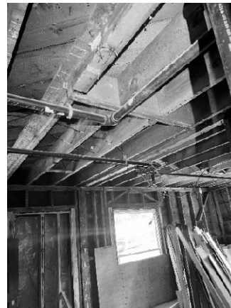
Figure 20 - Support for beam appears to be missing.
