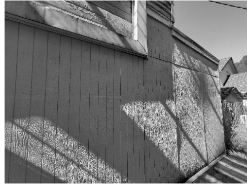
Figure 58 - Some of the siding panels have warped.
