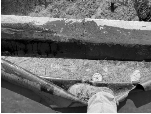
Figure 63 - Leading edge of EPDM membrane exposed roof assembly.
