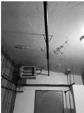
Figure 49 - In the kitchen add-on, there is black mold on the ceiling.
