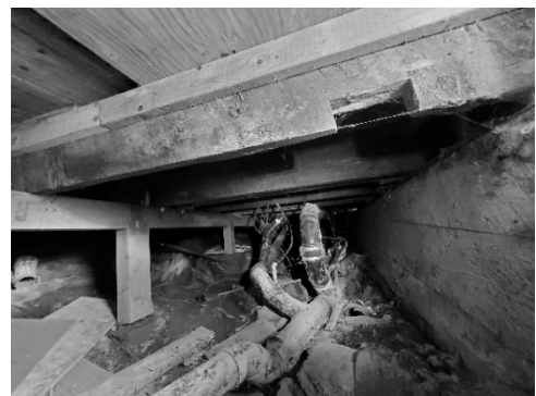
Figure 32 - Floor joist is notched in the crawl space.
