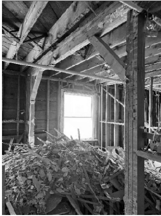
Figure 4 - Wall was removed, so diagonally braced walls do not stack.
