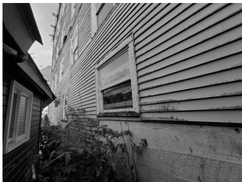
Figure 37 - Typical condition of exterior walls. There is potential rot at the window trim and siding where black mold is present.
