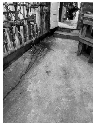
Figure 44 - The slab was cracked, and the floor was sloped.
