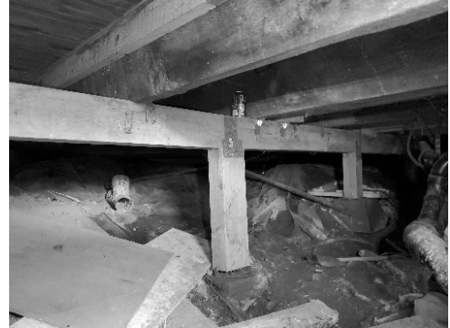
Figure 11 - One of the isolated footings has a corner that is undermined. Unknown if or how columns are connected to concrete footing.
