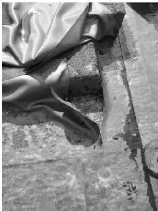
Figure 61 - Roof access hatch sheathing with water damage and shows signs of rot.
