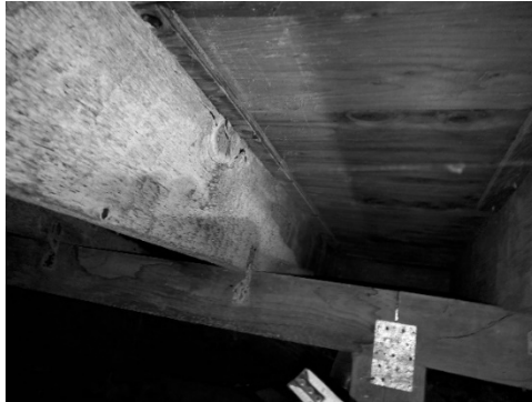
Figure 39 - Rotting joists along West side of the building near crawl space access hatch.
