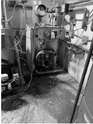
Figure 45 - There are signs of past leaks.
