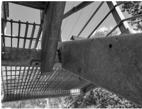
Figure 12 - There is a bolt missing from an emergency exit stair landing.
