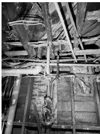
Figure 31 - The 1st level floor framing has a location where the diagonal boards are broken and appear to have been exposed to moisture.
