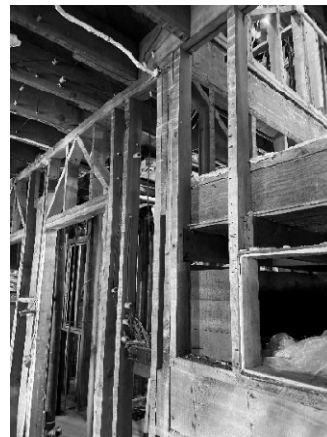
Figure 9 - No connection between beam and column.
