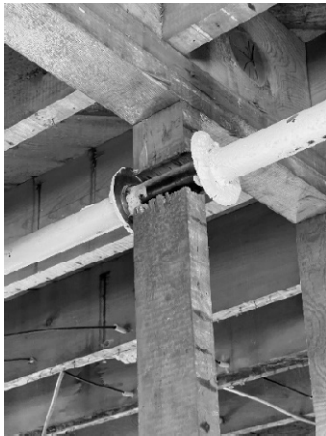
Figure 23 - Stud was cut for piping.
