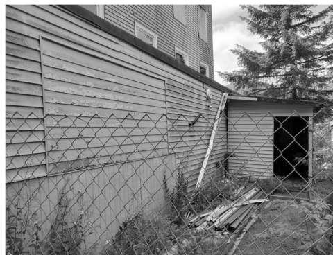
Figure 34 – Lower Shed Roof Failing
