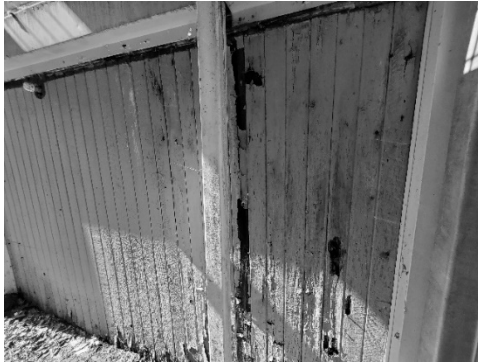
Figure 16 - Rotting T1-11 on the east side of the ground floor.
