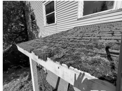
Figure 52 - There is significant moss on the entryway roof.
