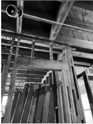
Figure 21 - Beam adjacent to stairway is bearing on a header.
