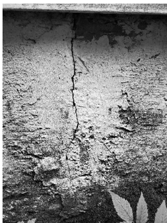
Figure 33 - There are a few cracks visible in the stem wall of the foundation.
