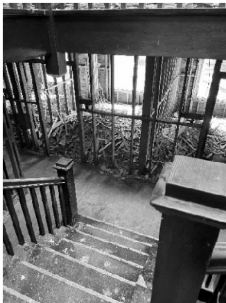
Figure 25 - Framing is long around stair opening with no intermediary support.
