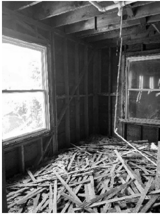
Figure 6 - Diagonally blocked exterior wall.
