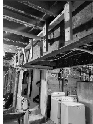
Figure 40 - Perforated steel beams supporting first-floor.
