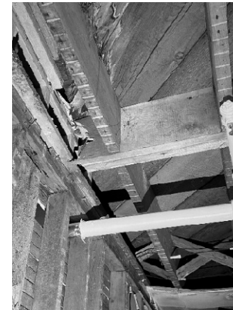
Figure 24 - Beam is broken.
