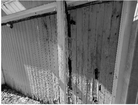
Figure 57 - In many locations, the paint is flaking.
