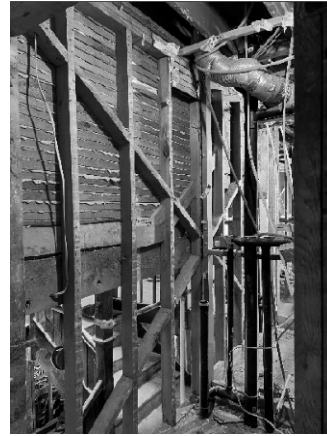
Figure 5 - Lath and plaster is on both sides of diagonally braced wall.
