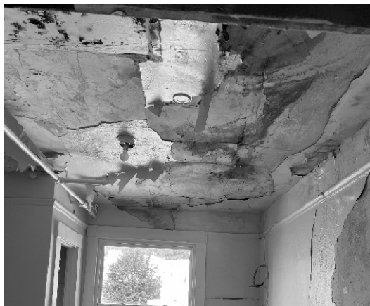
Figure 41 - Black mold and signs of water damage.
