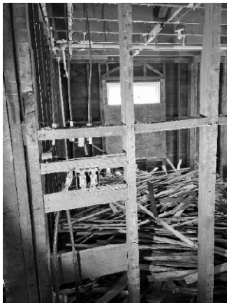
Figure 19 - Beam adjacent to stair opening bears on stud wall.
