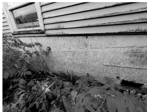
Figure 36 – Typical condition of concrete stem wall finish. Occasional crawl space vent penetration.
