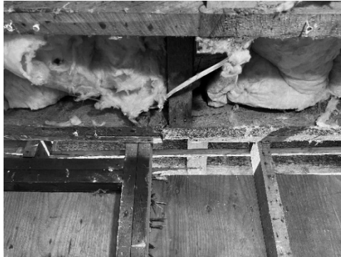
Figure 27 - A joist on the 1st level floor framing has a lot of deflection and is cracked.
