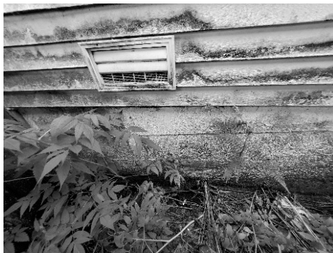
Figure 55 - Some of the exterior siding has black mold.
