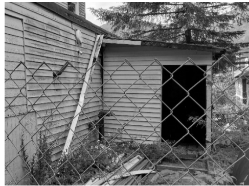
Figure 60 - The small shed on the back has significant moss on the roof, appears to have a roof leak, and is pulling away from the main building.
