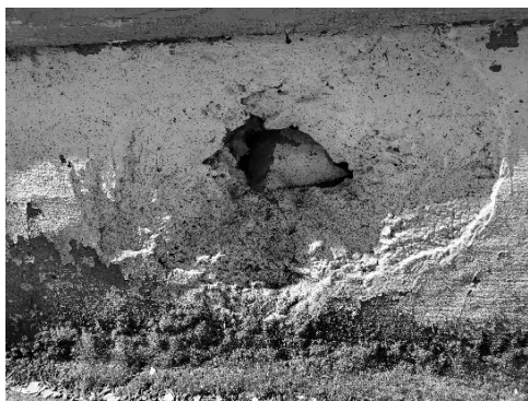
Figure 35 - Worst case of spauling found at the perimeter stem wall.
