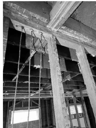
Figure 18 - Beam adjacent to stairway bears on stud wall, similar on all levels.
