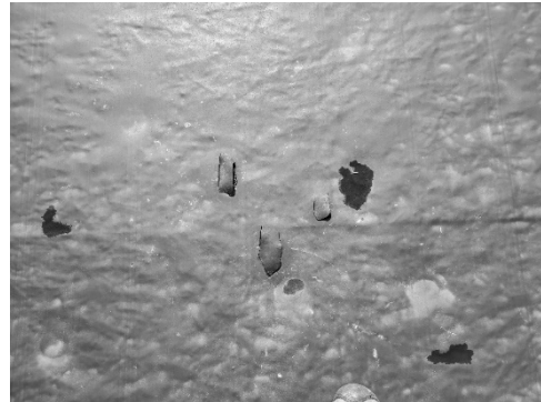
Figure 62 - Gouging in the roof membrane along the South side of the building.
