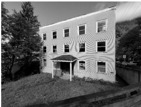
Figure 14 - The main entrance awning does not have lateral bracing.
