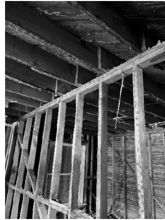
Figure 7 - Joist splice on wall is not blocked.
