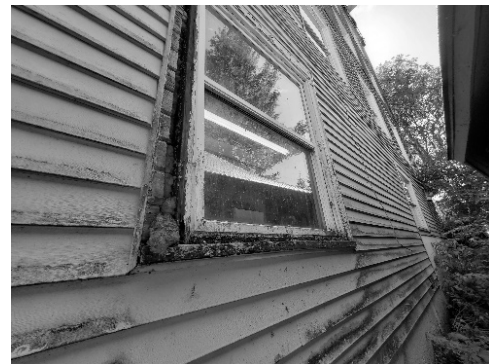
Figure 56 - This window does not have trim around the perimeter to prevent water infiltration.
