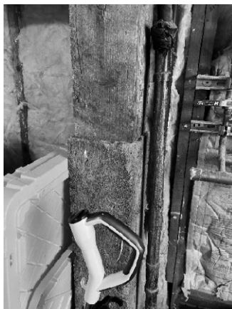
Figure 43 - There are no visible connections from the concrete pedestal to the column.
