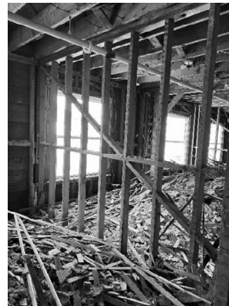
Figure 3 - Typical diagonally braced interior wall.
