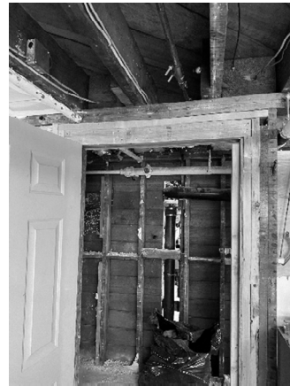
Figure 28 - The header has a lot of deflection and appears to be overloaded.
