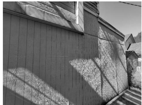
Figure 15 - New siding at the building addition warped and not fastened with enough nails.
