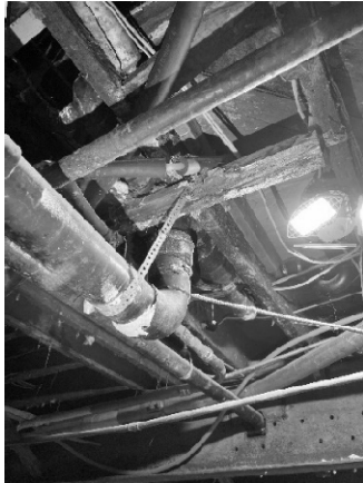
Figure 47 - There is a support board, holding up piping, that is rotten.
