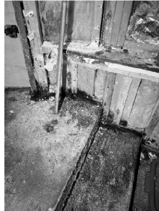
Figure 48 - There is mold at the interface between the wood framing and concrete stairs.
