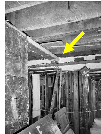
Figure 26 - Under the stairs, there is some framing with inadequate support.
