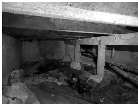
Figure 38 - New post-and-beam foundation for floor framing along West side of ground floor.
