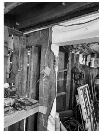
Figure 42 - There are no connections between post and beam.
