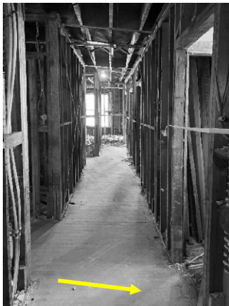
Figure 17 - Sloping hallway, similar on all levels.
