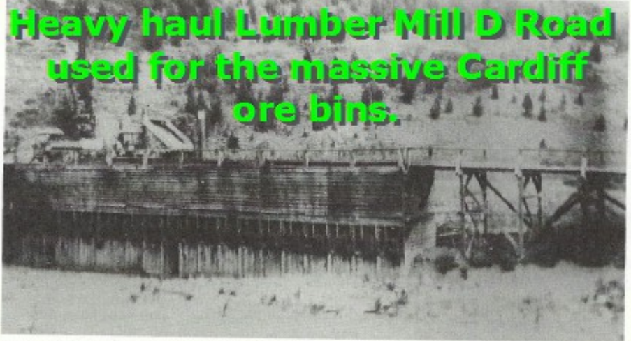
Figure 45. Cardiff ore bins located in Big Cottonwood Canyon at the mouth of South Fork. The company built these bins in 1916 to be used for temporary storage when motor vehicles replaced teams to haul ore down the canyon to the smelters. Company teams, and later trucks, brought ore from the mine to these bins. (UHS)
