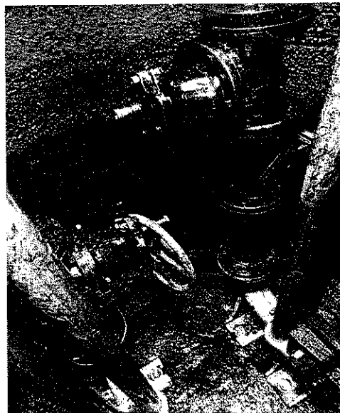
Picture 2: Existing discharge piping, check valves and isolation valves.
