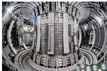
Interior of the JET Reactor with the ITER-Like Wall beryllium tiles installed
