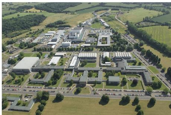
Culham Centre for Fusion Energy, Abingdon, Oxfordshire, UK
