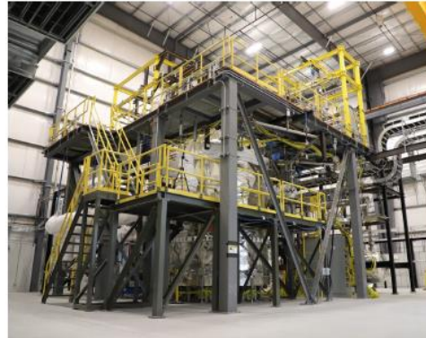
Construction complete / hot commissioning in progress November 2022
