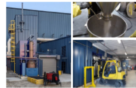
MSPP is located at the Materion Campus in Elmore, Ohio
