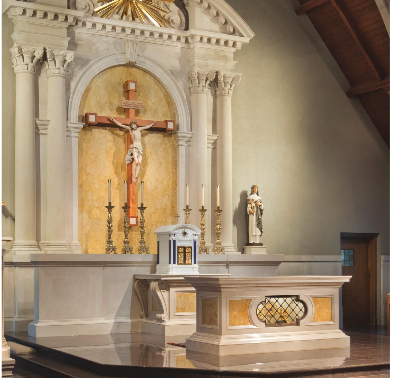
Drawing upon the existing geometry of the sanctuary triumphal arch, the new retablo stands more than 15 feet tall. On the retablo, four 12 1/2-foot-tall composite columns crafted from Indiana limestone surround a diamond-matched Giallo Reale marble niche and crucifix. The cornice and columns further support an upper stone pediment and volutes, which are also all constructed of Indiana limestone. Photo ©Duncan Stroik
