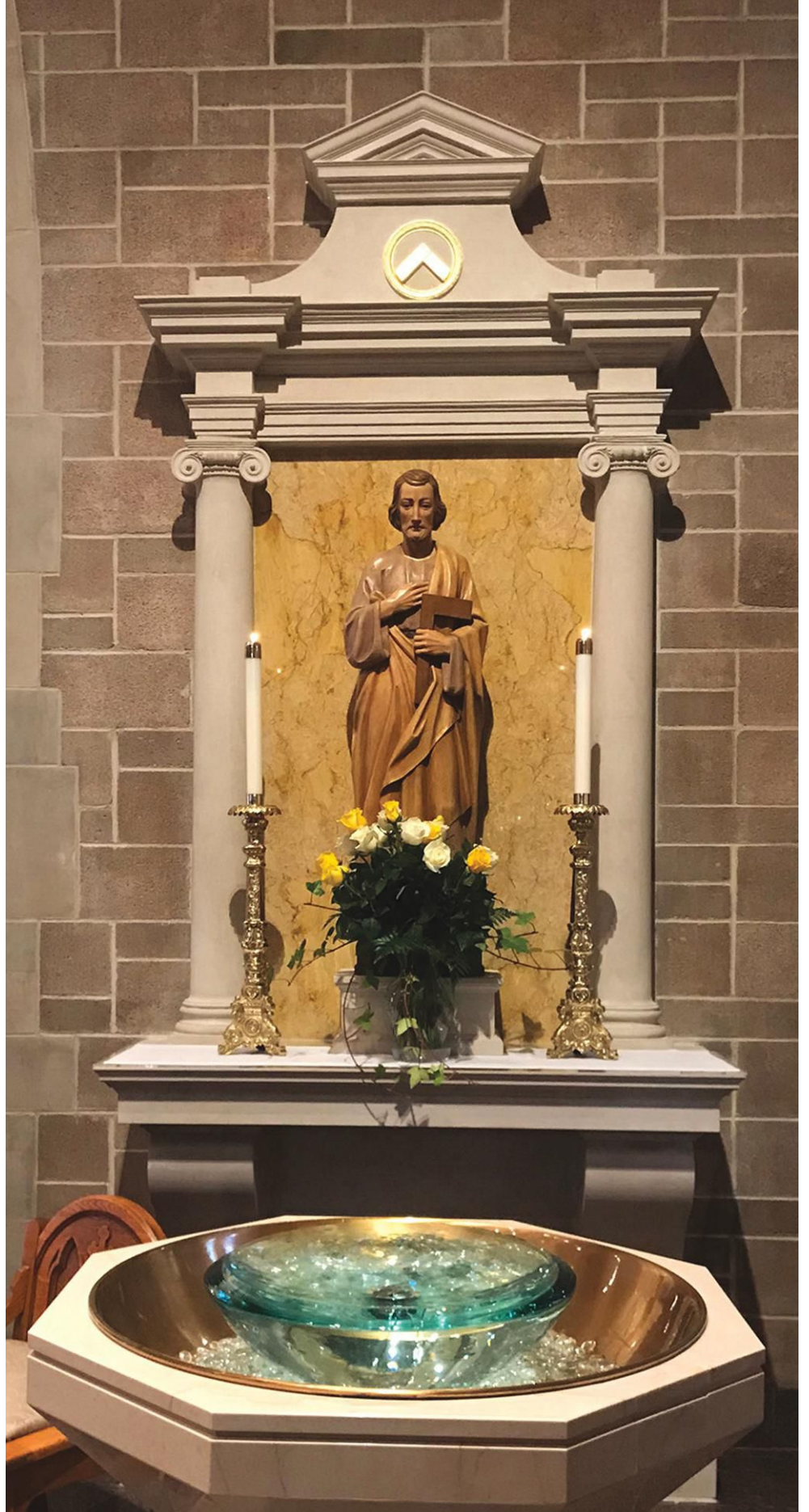
"Bookmatched Giallo Reale marble panels provide a backdrop for the two side shrine statues," Walton said. Photo ©Amy Mortensen
