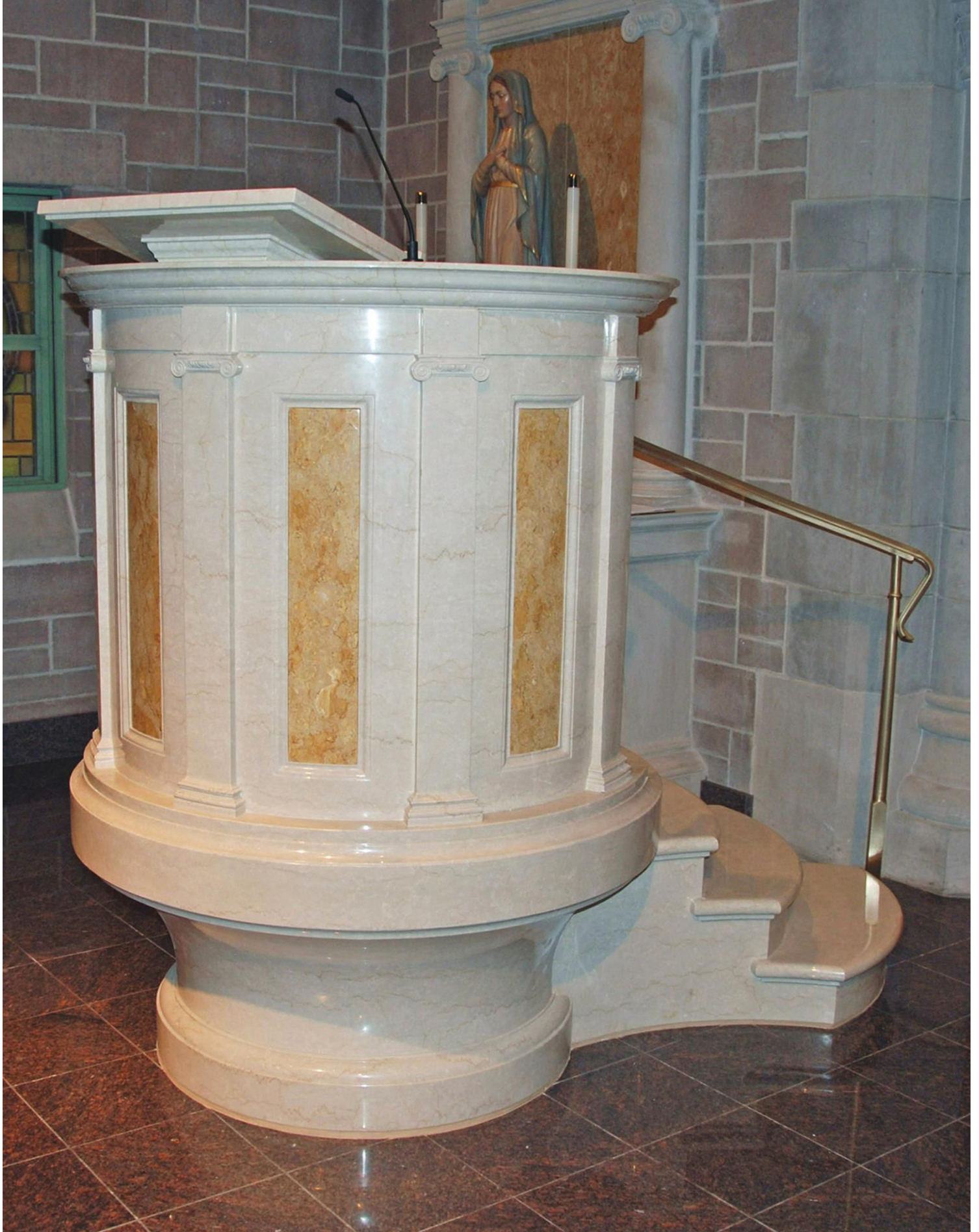
The cylindrical ambo was also reconstructd of Botticino Classico and Giallo Reale marble. Photo ©Duncan Stroik
