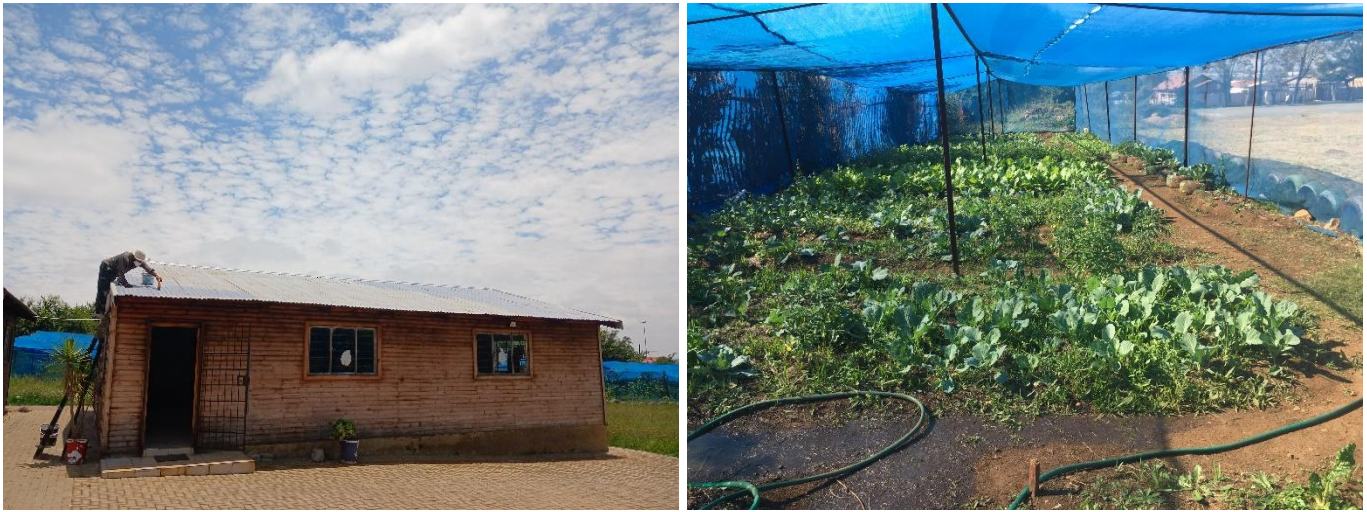
Building still needs restorative painting and garden shed now well restored
