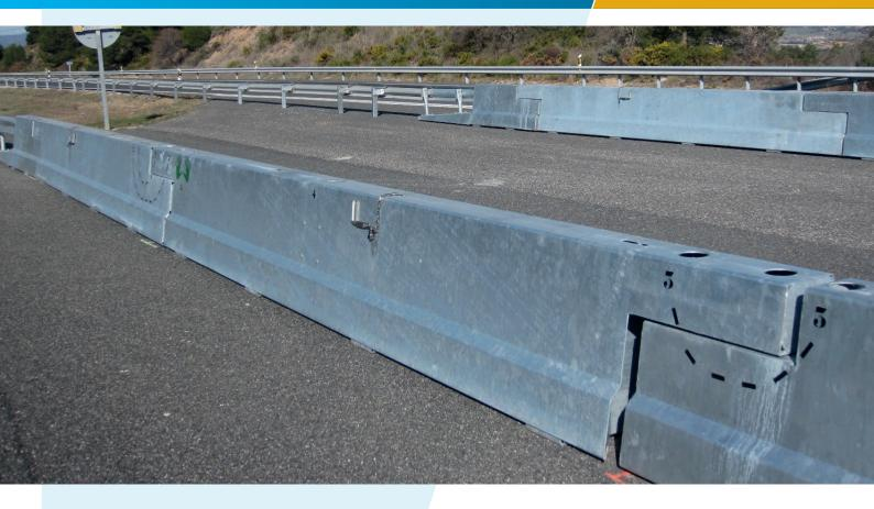
Openings in the central reserve guardrail or barrier are mainly needed as emergency gates, and in case of road works as gates to redirect the traffic to the opposite side. Opening gates are also indispensable in front of tunnels for emergencies or maintenance purposes. They can even be used as workzone access.
