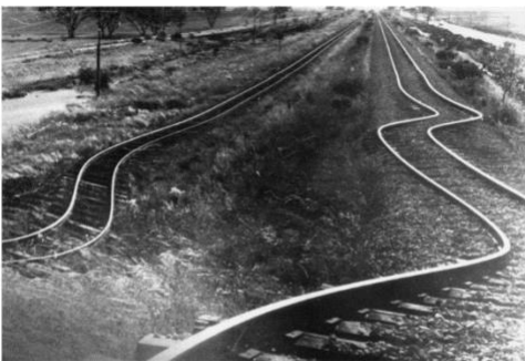
Railway after the Earthquake Meckering 1968
