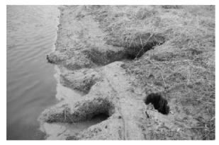
Figure 2. This neglected lagoon shows animal damage and poor grass care.
