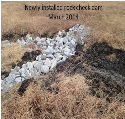
Newly installed rock check dam
