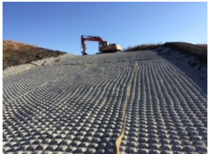
After flooding in 2019, this emergency spillway on a Little Walnut Hickory Watershed dam was repaired using a concrete mat. Funds were provided by the Watershed and through Emergency Watershed Protection Program funding available from the USDA Natural Resources Conservation Service.
