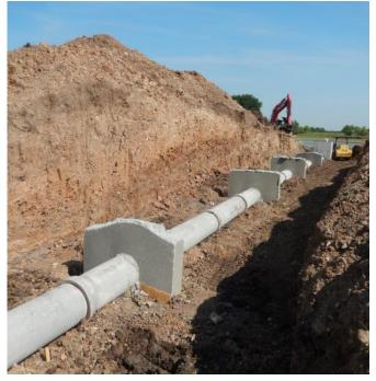
A principal spillway pipe replacement was completed in the summer of 2021 on a Whitewater River Watershed dam. The corroded corrugated metal pipe was replaced with a concrete pipe. The Kansas Department of Agriculture/Division of Conservation Watershed Rehabilitation Program provided cost share for the replacement.
