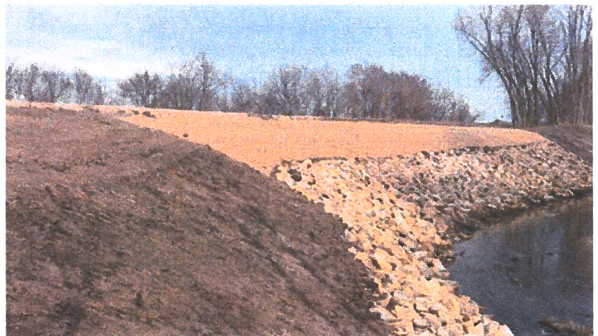
After the EWP exigency streambank stabilization.
