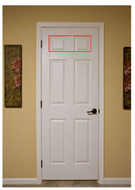
Measure the width and height of the cut out you will make in the door as shown by the red lines. The cut out should be at the edge of the flat surface of the door on all 4 sides of the panel.
