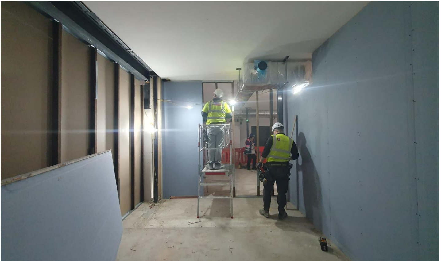
Image: completed installation – Acton, London, UK (Feb 2026)
