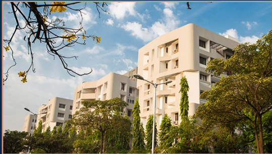
Landmark Garden Phase-2 Kalyani Nagar, Pune | 2011
