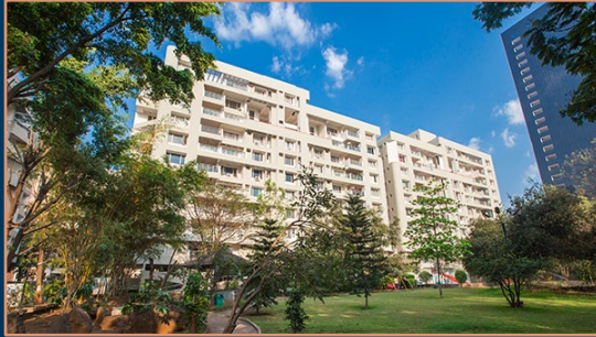
Landmark Garden Phase-1 Kalyani Nagar, Pune | 2001
