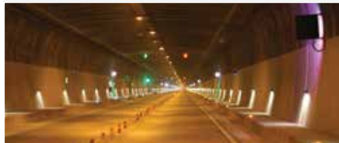
2017 Chenani-Nashri Tunnel, Jammu & Kashmir
