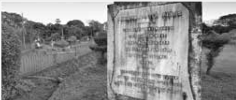
1887 Malabar Hill Reservoir, Mumbai
