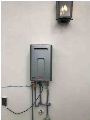
Gas Water Heater
