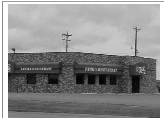
Sign, Architectural Canopy Sign, Awning or Canopy
