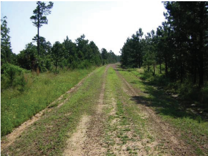
Figure 7. Crowned Road with Ditches.
