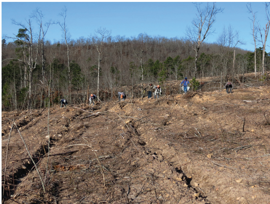
Figure 23. Ripping on Contour.
