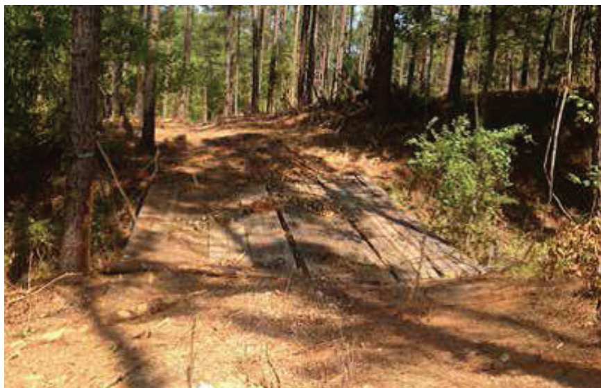
Figure 19. Portable Bridge Mats.
