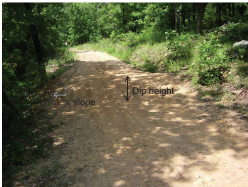
Figure 12. Example of a Rolling Dip.
