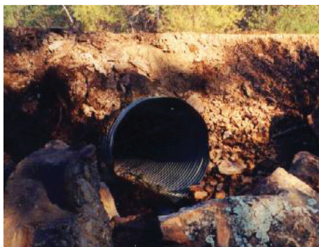
Figure 10. Cross-drain Culvert with Armored Outlet.
