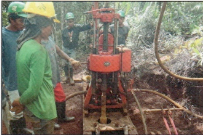
Figure 7.1.2: YHP drill machine in operation
