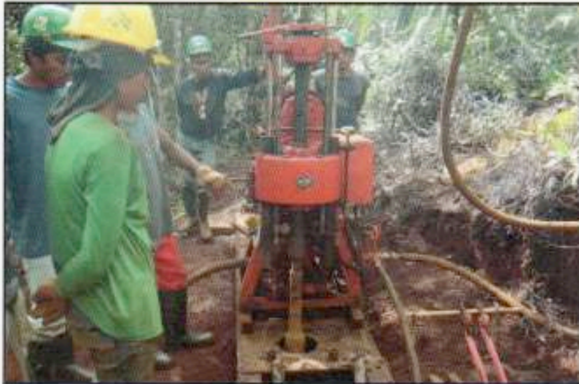
Figure 7.1.2: YHP drill machine in operation
