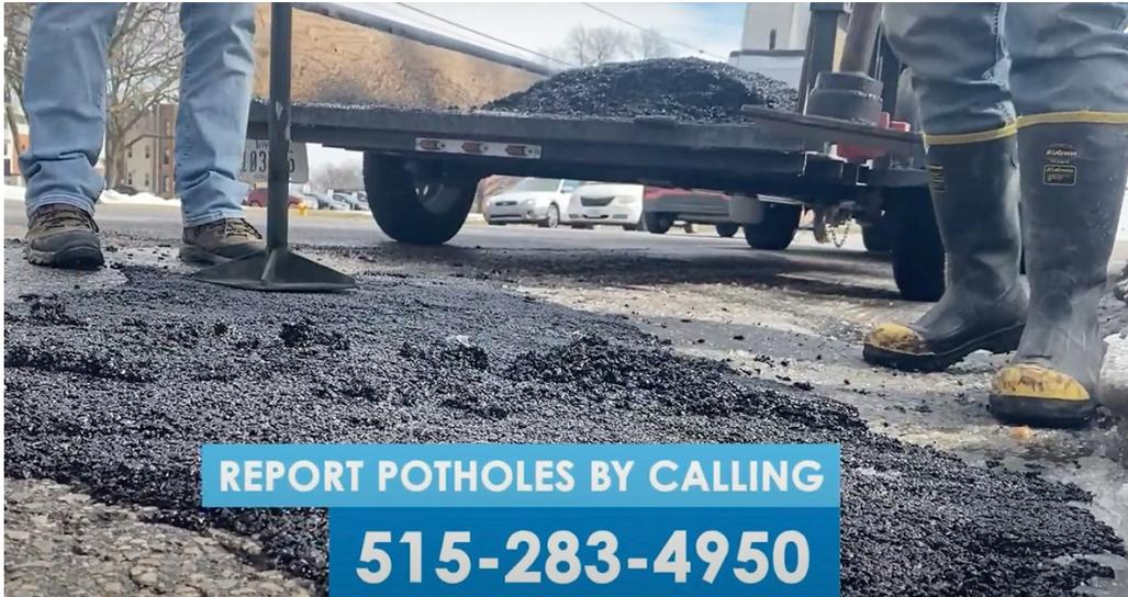
With these drastic weather changes this month, we are entering pothole season earlier than usual. The freezing temperatures and snow followed by warm weather causes the ground and road to shift, resulting in increased potholes.
