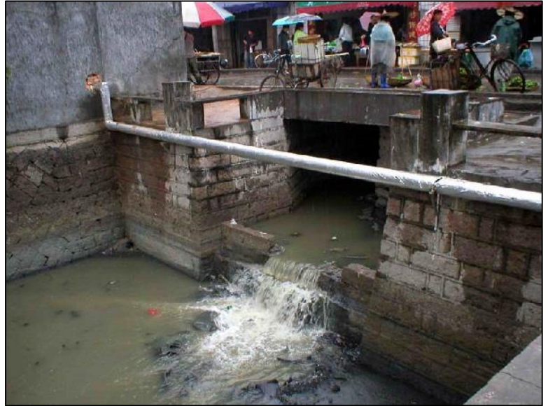
Raw sewage entering into the canal
