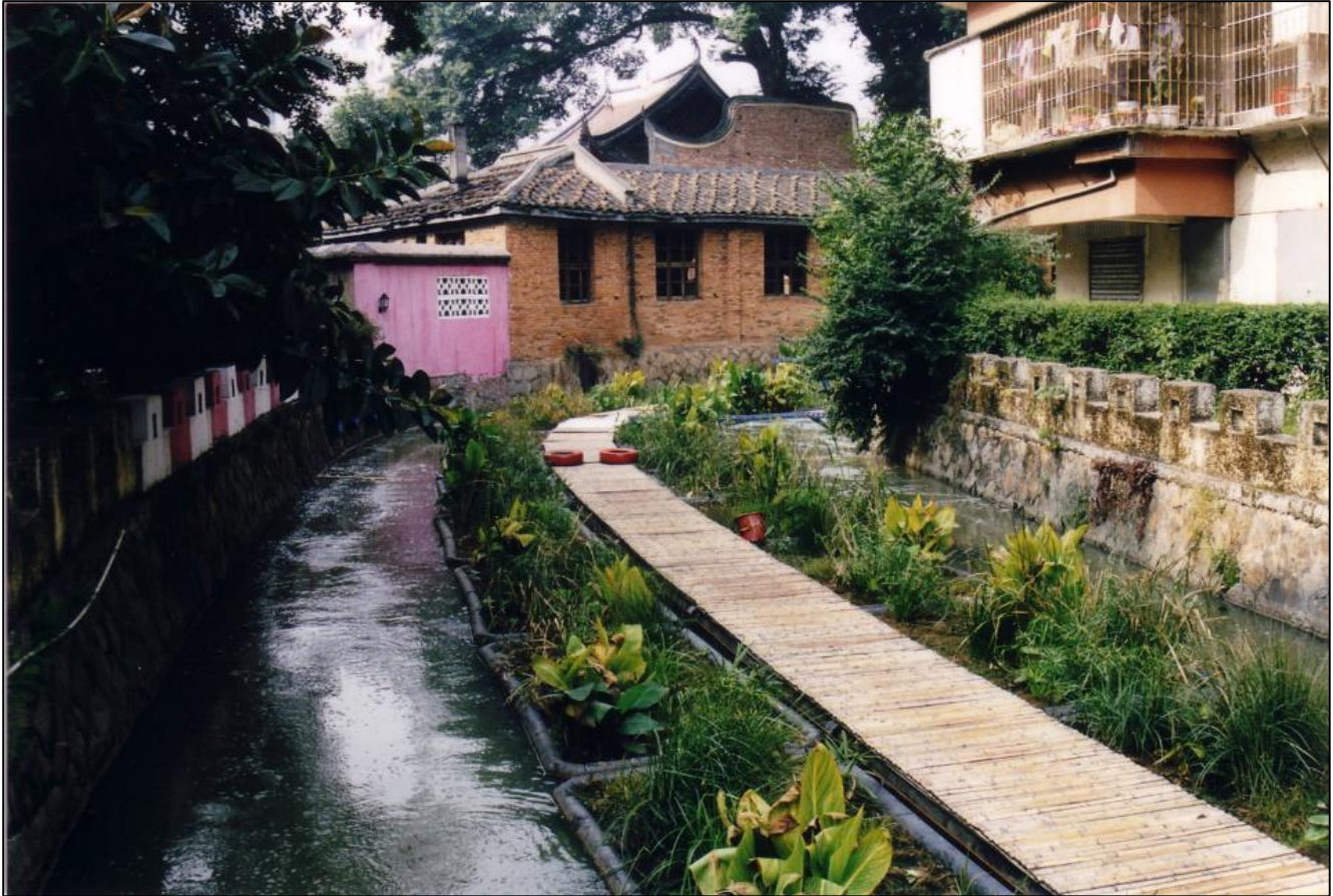
The Baima Canal with a Restorer system remediating contaminants out of the canal
