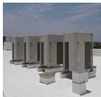
Variable Refrigerant Volume (VRV)
