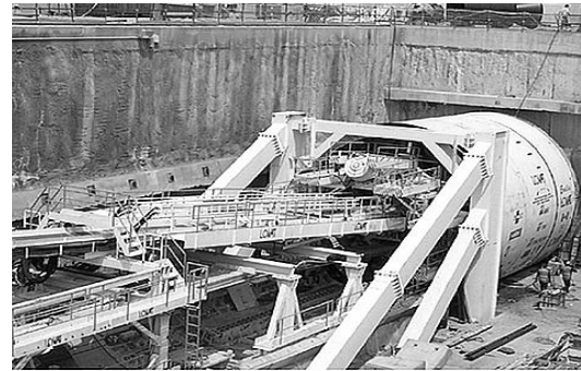
Figure 4-2. EPBs used at the Bologna – Florence project
