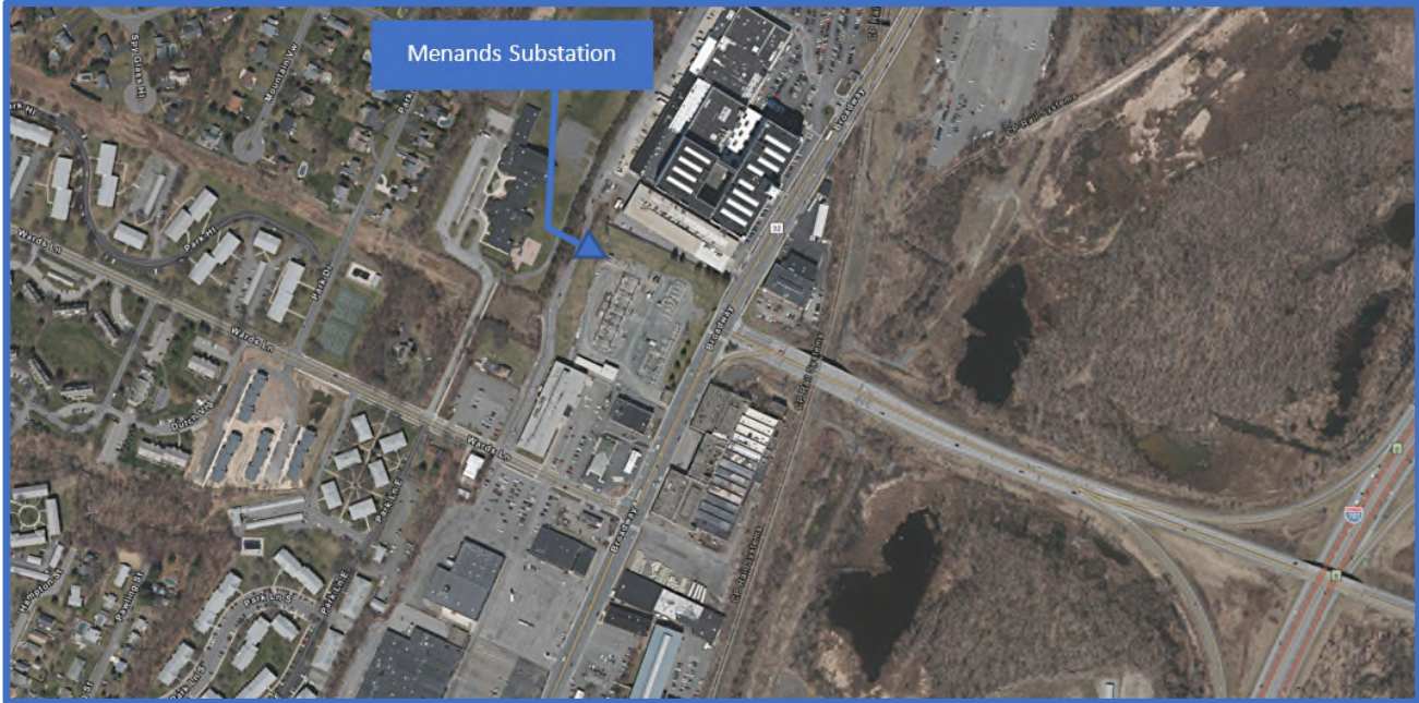
Figure 14: Satellite view of Menands Substation within the City of Albany near the intersection of Broadway and Wards Ln.
