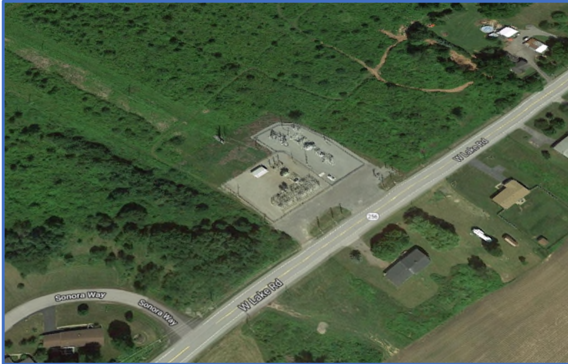
Figure 9: North Lakeville Substation (left) and Sonora Way Distribution Substation (right)
