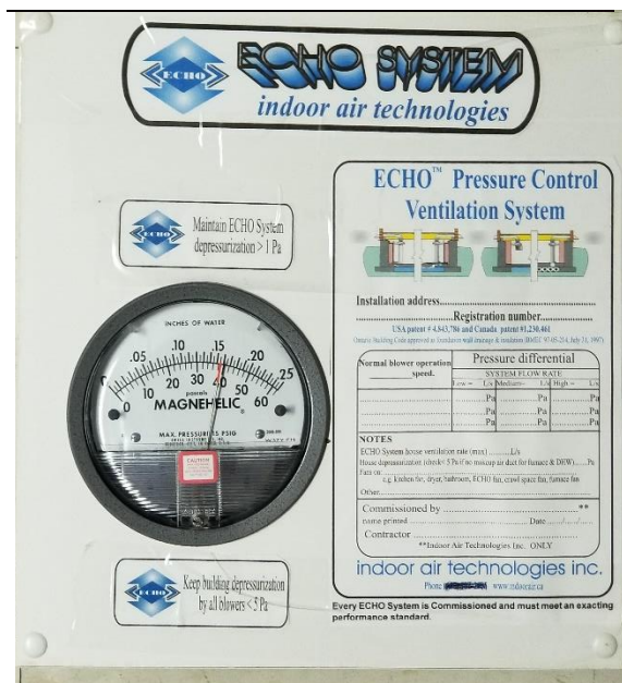
Figure 3 The ECHO System Control Panel with the differential pressure meter, the blower speed control, the connections to pressure sensing tubes and the commissioning certificate.
