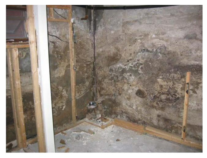
**Stone foundations** are major sources of basement dampness and mold growth in the stone interstices. Finishing such basements with the ECHO System produces major basement air quality and comfort improvements.
