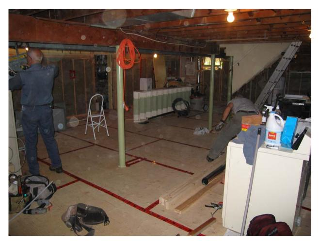
**Ventilated ECHO subfloor.** The ECHO sealed and ventilated subfloor is less than 1-3/4" thick. Two thirds of the floor cross section comprises a low emissivity air cavity. Water can safely flow through this cavity to an interior drain if there is extensive foundation water leakage or a flood.
