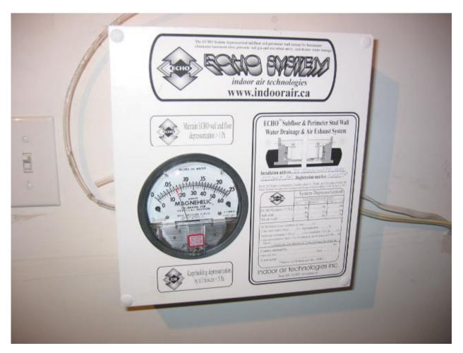
The ECHO System control panel provides the System registration number assigned by Indoor Air Technologies to the Commissioned system. It contains the ECHO blower speed control and the pressure differential monitor. The pressure indicator in this photograph shows an ECHO System depressurization relative to the basement air of 16 Pascals. This depressurization is more than adequate (2 Pascals is adequate) to remove concrete 'rising damp' and soil contaminant gases.
