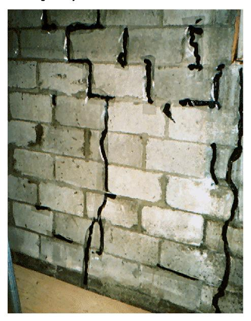
**Concrete block air leaks.** These porous foundations provide sites for mold growth and a network of passageways for water ingress and soil gas entry to the block cavities, and multiple small openings into the basement and upstairs, drawn in by building stack pressures. Stack pressures act whenever the house is warmer than outdoors. ECHO System coverage can offset these stack pressures and eliminate this avenue of contaminant entry through porous grout fillings.
