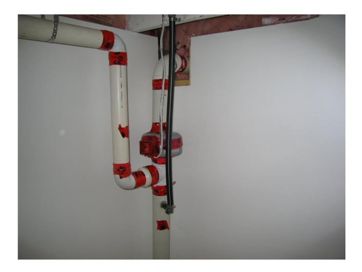
**ECHO Blower, PVC piping and sump tube.** The complete perimeter stud wall and subfloor assembly is exhausted to the outside by a continuous duty blower. The System is pressure-tested and leaks sealed before drywall installation. This ensures complete venting of the wall-floor assembly at the lowest possible exhaust rates for the System layout and foundation type.
