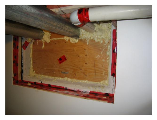
Crawl space hatch with HVAC ducts and ECHO exhaust duct (white PVC). Crawl spaces with dirt floors are a principal source of house air fungal spores and gases. The ECHO System can be used to eliminate this problem.
