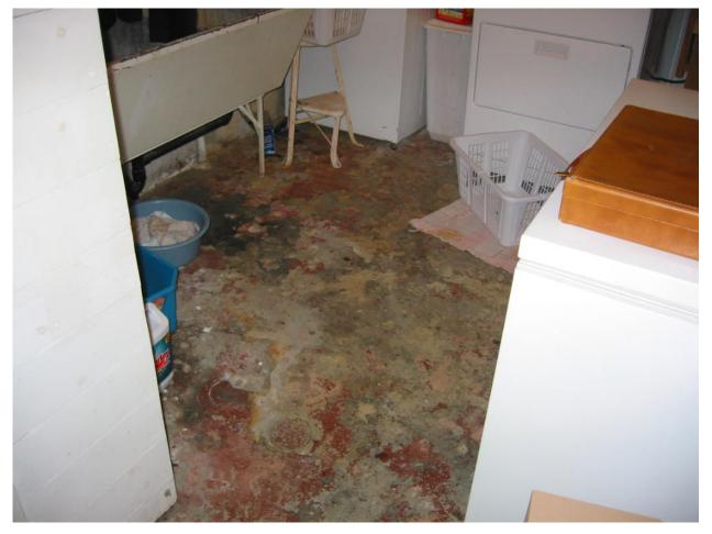
Concrete capillary moisture – 'rising damp' causes paint peeling. Basement moisture problems include peeling foundation and floor slab paint, white concrete efflorescence, visible and hidden mold growth, and the typical basement odor.
