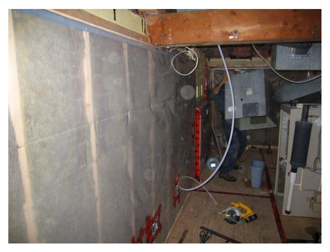
**ECHO Wall.** The ECHO sealed and ventilated stud wall is fully and tightly insulated, and the normal insulated stud wall thickness of 4 inches. However, unlike normal insulated walls, ECHO walls do not have energy robbing convection currents and damp insulation. In the ECHO wall, controlled ventilation keeps insulation dry and any water ingress or condensation can safely run down the foundation wall behind the insulation to the floor where it is quickly ventilated and/or drained away.
