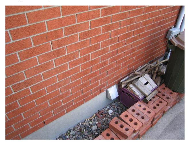
**The ECHO System exhaust** is vented outdoors like a dryer vent. The ECHO System exhaust air temperature is typically ~ 15C (60F), so it will melt nearby snow in winter, and provide energy savings for a nearby air conditioner or heat pump.
