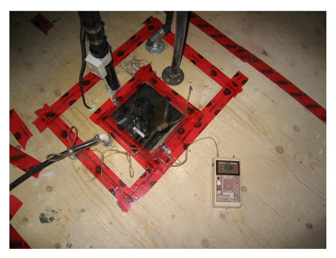
**Basement sumps** are a principal source of house air contaminants. Their water, if stagnant, becomes a microbial amplification site. The pipe(s) into the sump from perimeter foundation weeping tiles inject soil humidity and gases such as radon and microbial VOCs and spores into the sump and from there into the house air itself. The ECHO System eliminates this problem by venting the sump air directly to the outdoors.
