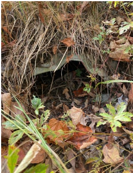
Inlet (left) and outlet (right) of crushed culvert across River Road. Right photo also shows erosion of channel.
