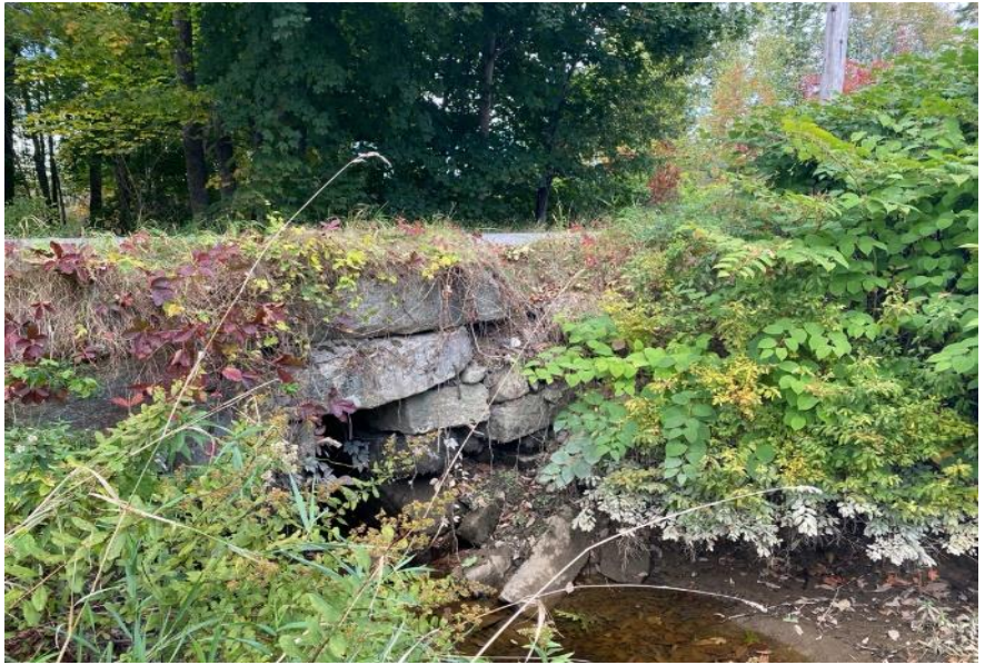
Culvert at crossing outlet with failing wall.
