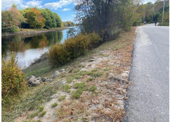
Road shoulder erosion and rocks dumped adjacent to the Narraguagus River.
