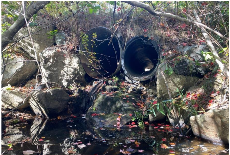
Twin culverts along Stillwater Road with perched outlets.
