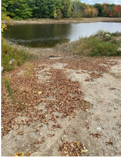
Left: Sheet erosion along boat launch going into river. Right: Erosion on Wilson Hill Road washing sediment down the boat launch access road.
