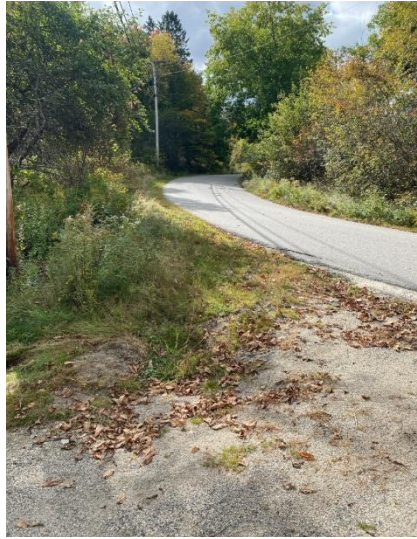
Left: Sheet erosion along boat launch going into river. Right: Erosion on Wilson Hill Road washing sediment down the boat launch access road.
