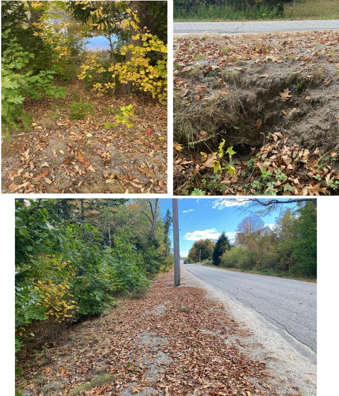
Top Left: Erosion leading down to the Narraguagus River. Top Right: Crushed culvert and unstable outlet. Bottom: Excess winter sand along River Road.
