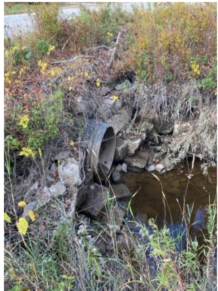
Left: Streambank erosion along the tributary. Right: Perched culvert outlet and deteriorating wall.
