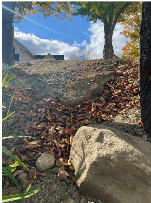
Left: Culvert filled with sediment. Right: Erosion coming off River Road adjacent to the culvert.
