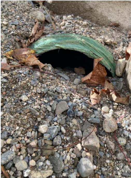
Left: Culvert filled with sediment. Right: Erosion coming off River Road adjacent to the culvert.
