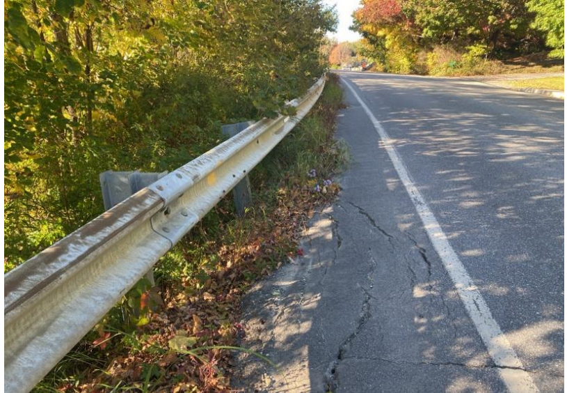
Photo shows cracking and slumping of road from stormwater.
