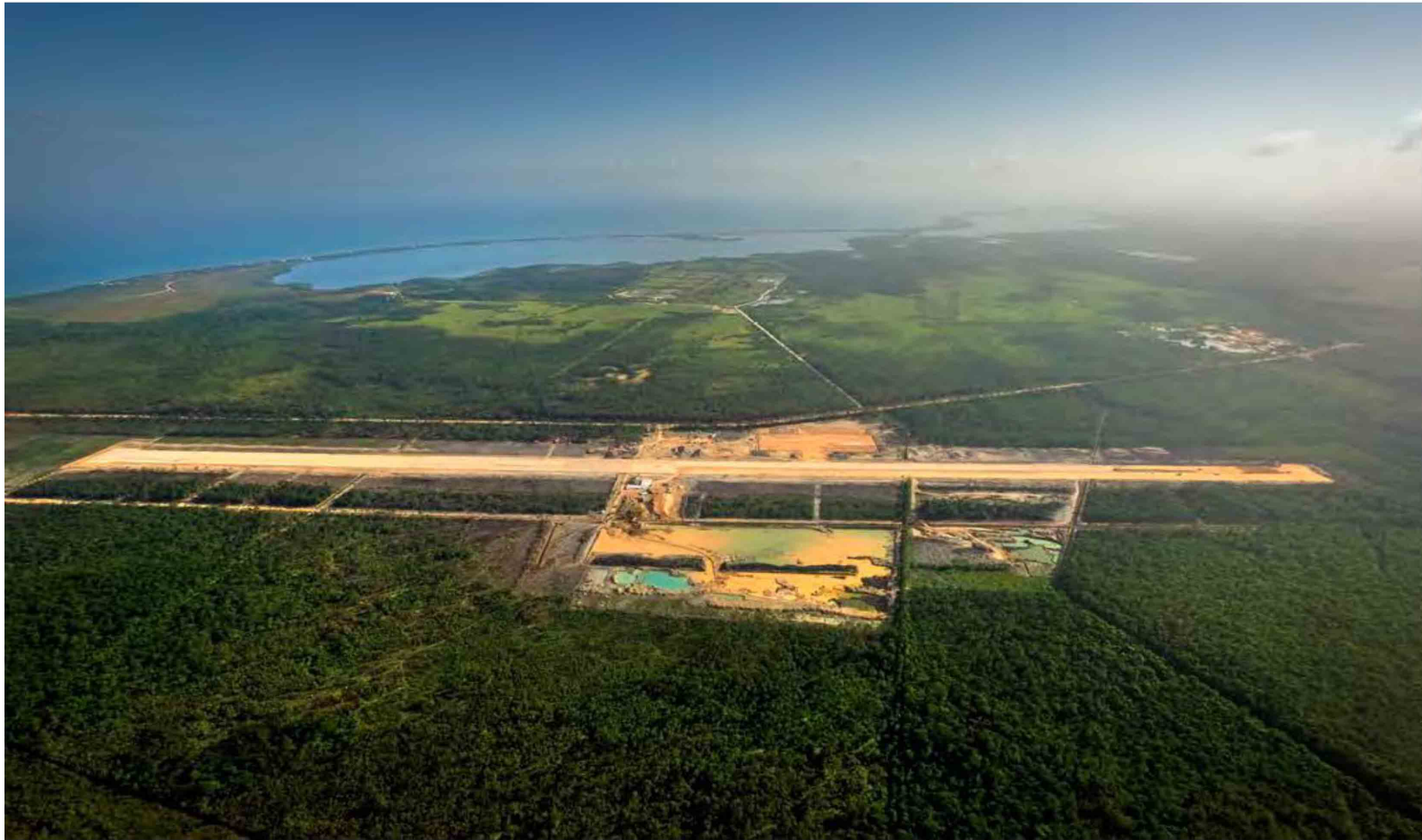
Construction at Placencia International Airport – 9200 foot runway
